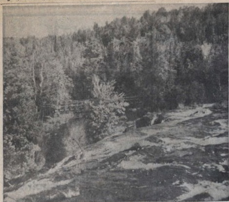
BOND FALLS recreation area offers many vacation and holiday opportunities for tourists and local residents. The rustic bridge shown here is one of the many improvements made to the site to enhance natural attractions found on this U.P. Power Co. property. Fishing here is excellent.
