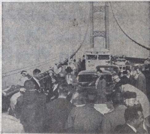
Government, science and labor get together at the bridge opening. Here Michigan's Governor, G. Mennen Williams, at left, is talking with the bridge builder, Dr. D. B. Steinman, and "Big Louie" Stepmann, a bridge employe who made headlines when he survived a fall from the bridge.
