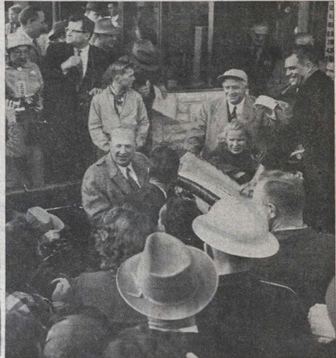
After nearly 3 years abuilding, traffic starts moving across the Mackinac Straits bridge. Prentiss M. Brown, chairman of the Bridge Authority, is pictured above selling first toll ticket to Governor G. Mennen Williams on Nov. 1, 1957. The event capped the huge construction project and marked the first step toward refunding the bonds which made financing of the bridge possible.
