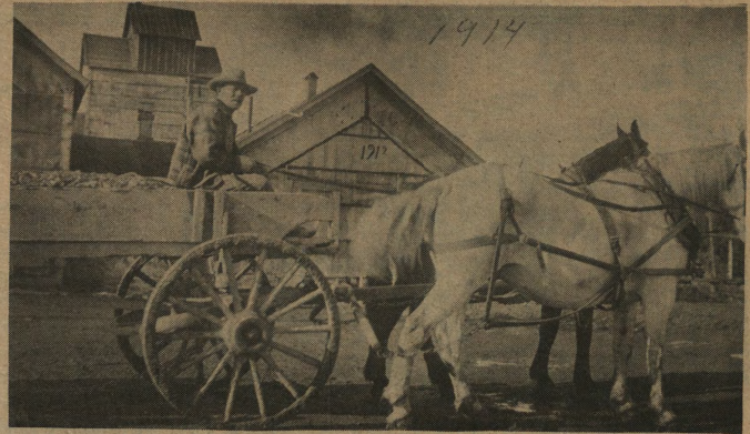
#3 ROCK HOUSE & "DRY", WHITE PINE, BUILT IN 1912. AARO SAVOLA SR. IS THE TEAMSTER HAULING ROCK.
