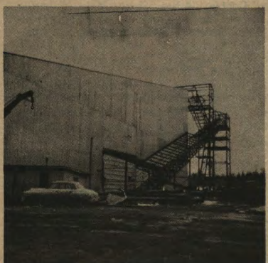
SOUTH END MILL BUILDING AND THE CONSTRUCTION OF C9 CONVEYOR
