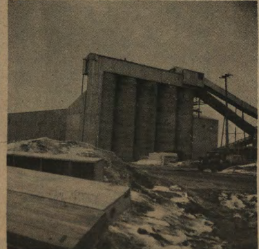
ORIGINAL 5 CRUSHER BINS AT W.P. MINE
