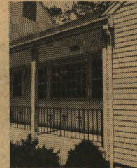
SOLID VINYL soffit and fascia systems supplement the line of horizontal and vertical sidings. Solid vinyl gutters and downspouts, including all accessories, are also manufactured by Bird & Son, Inc., East Walpole, Mass. They can't peel or blister like wood, or corrode, pit or dent like metal.
