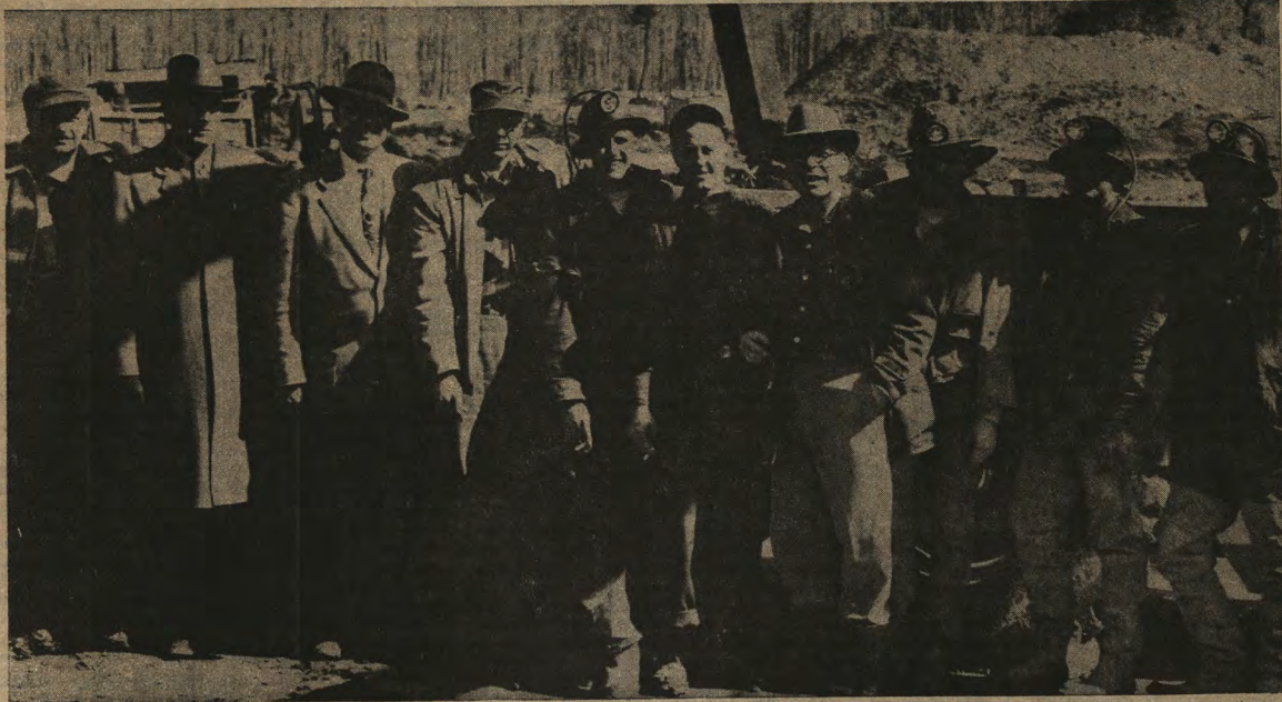
—Gazette Photo THESE men aided in the achievement of Tuesday's event at White Pine . . . the bringing up of the first load of "pay dirt" (copper ore) since the project was started. (L to R)—Edwin Bennett, Turner Construction Co. superintendent; George Reaves, Turner Project Manager; Harold Ewoldt, vice-pres., White Pine Co., Charles Haberlen, chief mining engineer; Harold Raymond, mining engineer; Richard Mansfield, maintenance engineer; Gerald Warrenner, resident engineer, White Pine Co.; Larry Garfield, mining engineer; Gervase Smith, miner and Bernard Chaput, miner.
