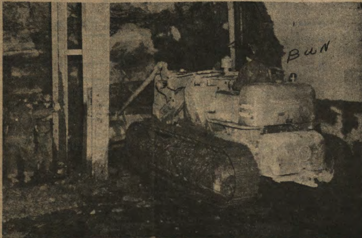
SETTING STEEL—Steel supports for the roof of the main service drift were being set near the collar of the drift when this photograph was
