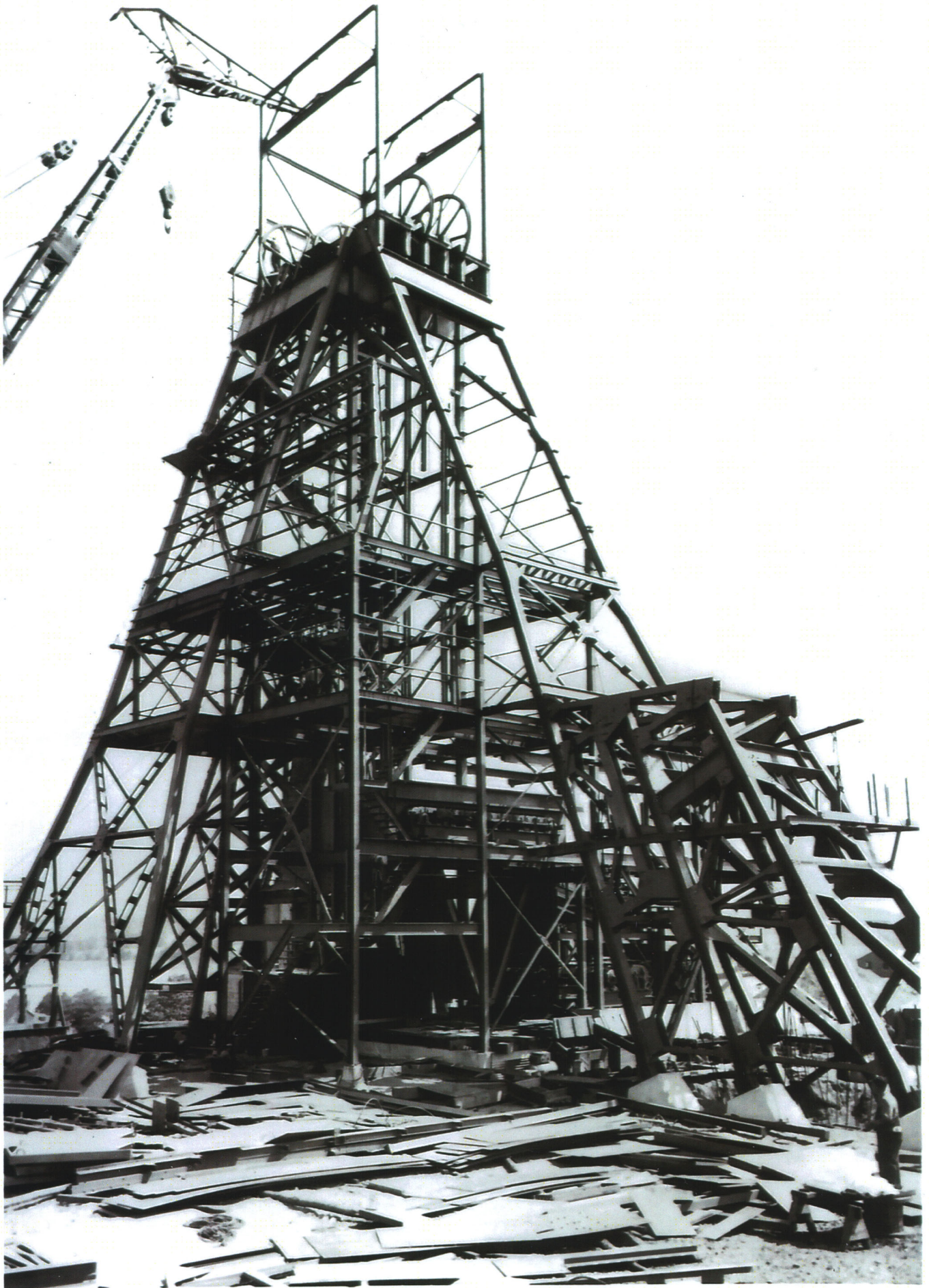
Mather R Mine Shaft Construction Looking Northeastly
