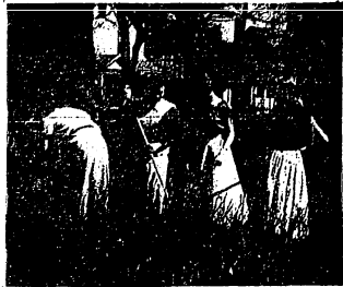
CLEANING HIGH SCHOOL YARD
