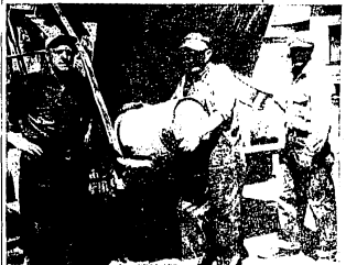
CITY CREWS ON THE JOB
