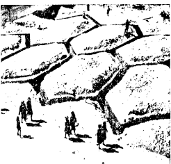
The old trenches that set up an area "more alive in Italy" in a waffle-like pattern are being used by the Wehrmacht divisions near the headquarters of the 13th Air Force in Italy. This new type of trench is said to offer considerable more protection, and is harder to hit from air.
