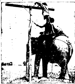
A member of the American signal construction squad is shown raising a line from the back of an elephant. Three new-made, black animals are used to very good advantage in the swamps of Alaska. By means and other things, the signal corps, under actual conditions, has managed to install and keep up communication lines.
