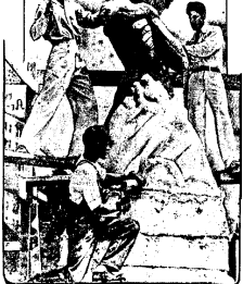
The Public Works Administration work of an project was being...
