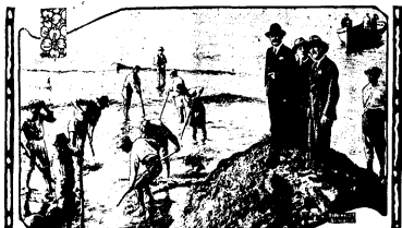
The new direct cable between Italy and America has just been laid. This photograph, just received from an above workman attending the submarine cable in the Corrienti-Orfagna line off which connects with Rome.
