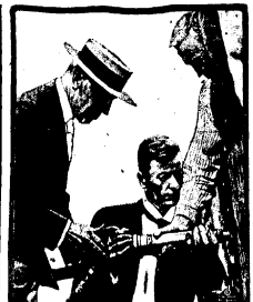
President Wilson is here seen driving the first rivet into the hull of a 10,000-ton cargo steamer, this being the first boat to be laid by the steel shipyard at Philadelphia, Pa.
