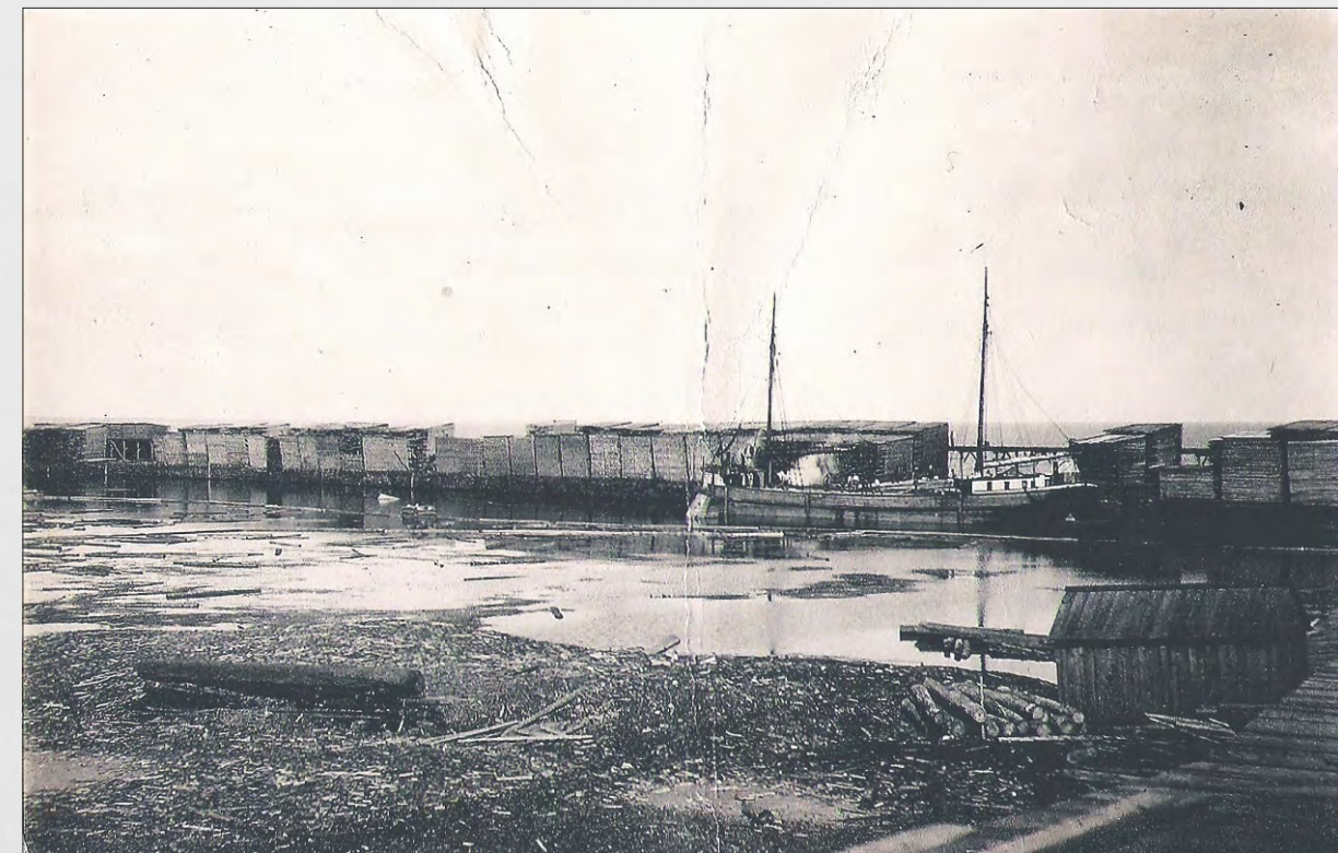
The Delta Lumber Company created a pond of several acres into which logs were stored prior to being milled. The pond could hold at least 8 million board feet worth of logs and was also utilized as a safe haven for boats during bad weather.
