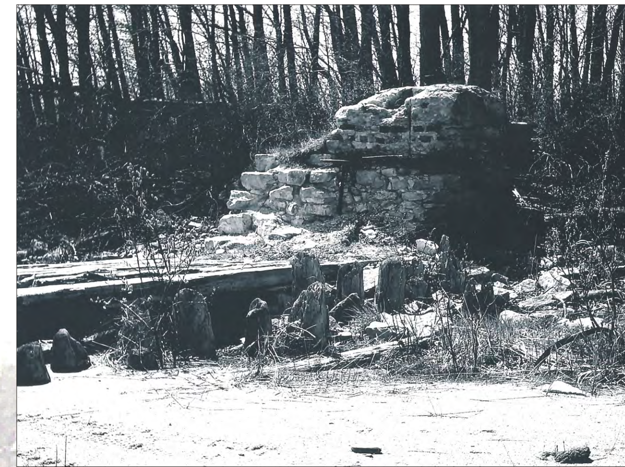
One of the few remaining signs of the Mill is the crumbling foundation of the power plant. In the spring dock pilings can also be seen along the old shoreline and out into the lake.
