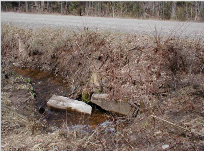
Site #11 - Reany Creek/County Road 510 culvert replacement ('08).
