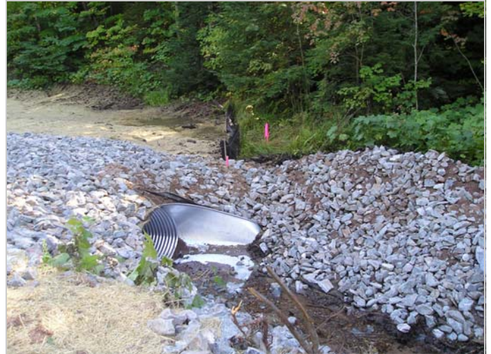
Site #11 - Reany Creek/County Road 510 culvert replacement ('08).
