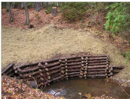
Photo of cribwall installation on Nordwald Creek, October 2008
