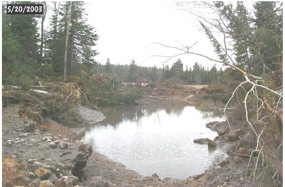
CR AAT washed out at Mulligan Creek crossing.
