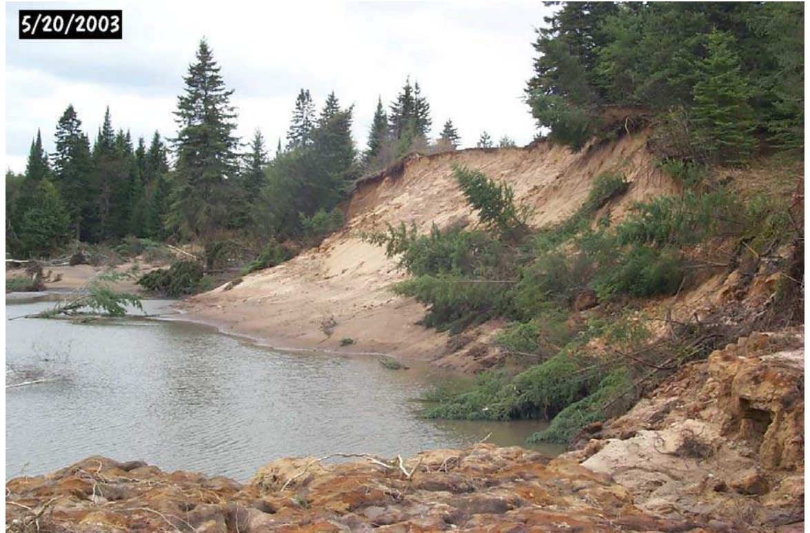
Large scour area along the Dead River washed out CR AAT just upstream of the Mulligan Creek bridge crossing. Next photograph is a view from the top of the bluff, which is the former location of CR AAT.
