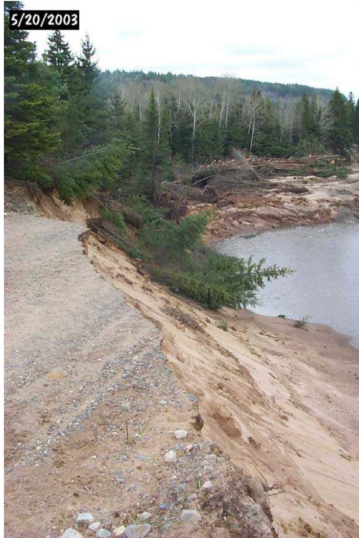
View from the top of the bluff seen in the previous photograph showing the large bank that was washed out in the 2003 Dead River flood event and what is left of CR AAT on the left of the photograph.
