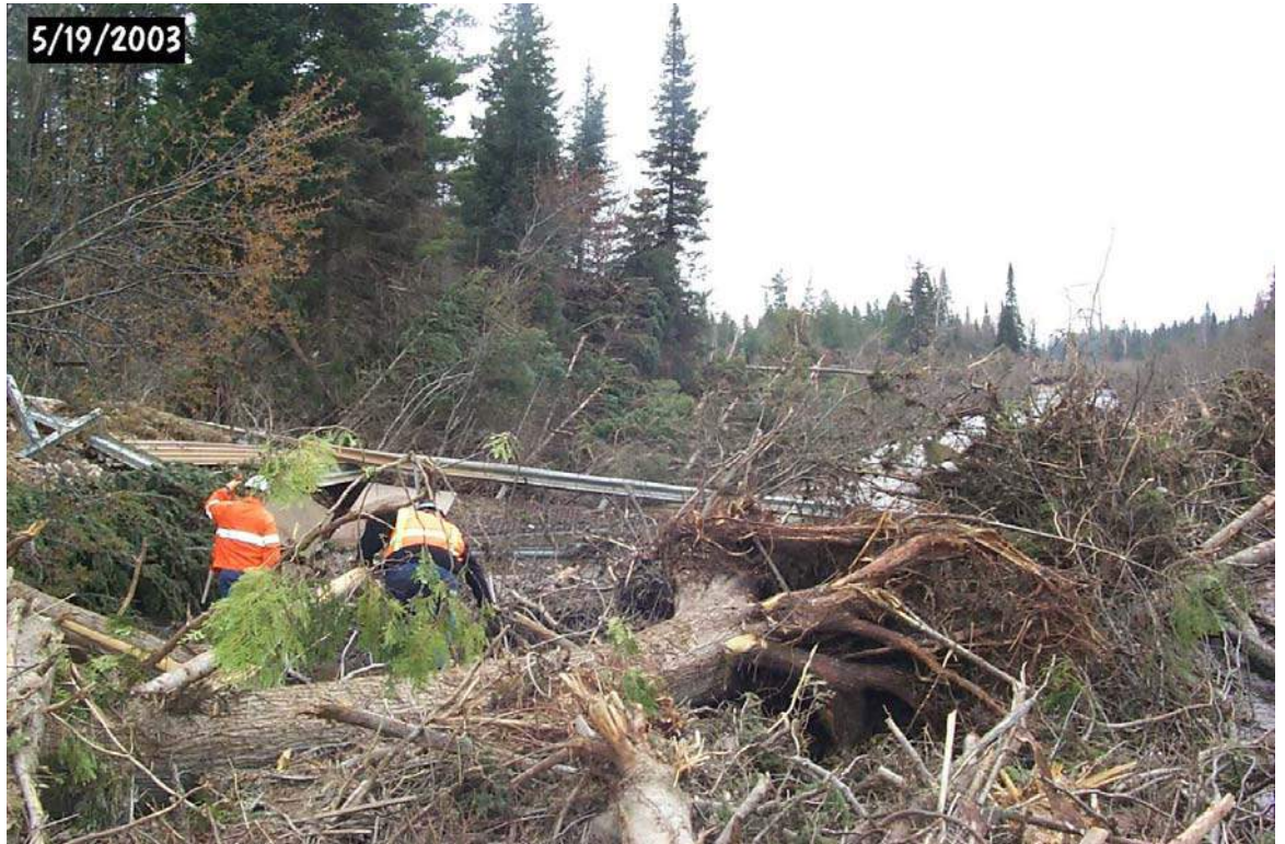
Remnants of the former bridge over the Dead River at CR AAO.
