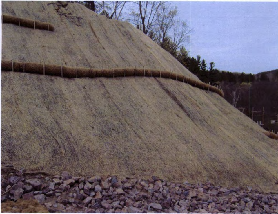
RM-10 looking north (North side of corridor)
