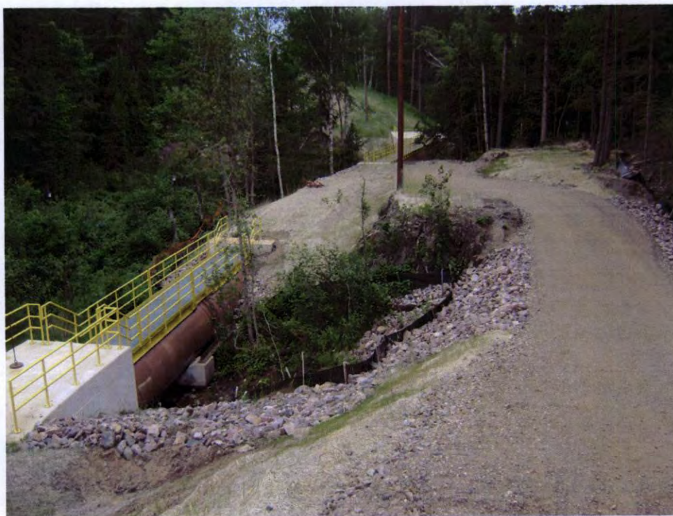
RM-9 looking northeast (South side of corridor)
