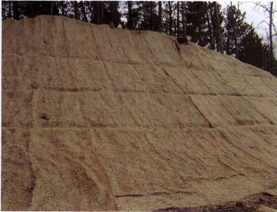
RM-10 looking north (North side of corridor)
