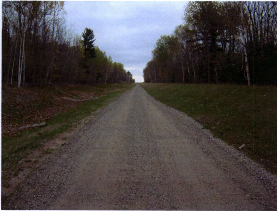
Overall site vegetation between RM-4 and RM-5 (Looking down-stream of penstock flow)
