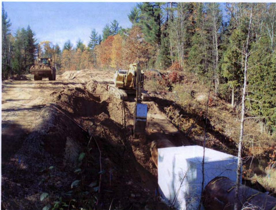
Rough grade being completed near RM-9
