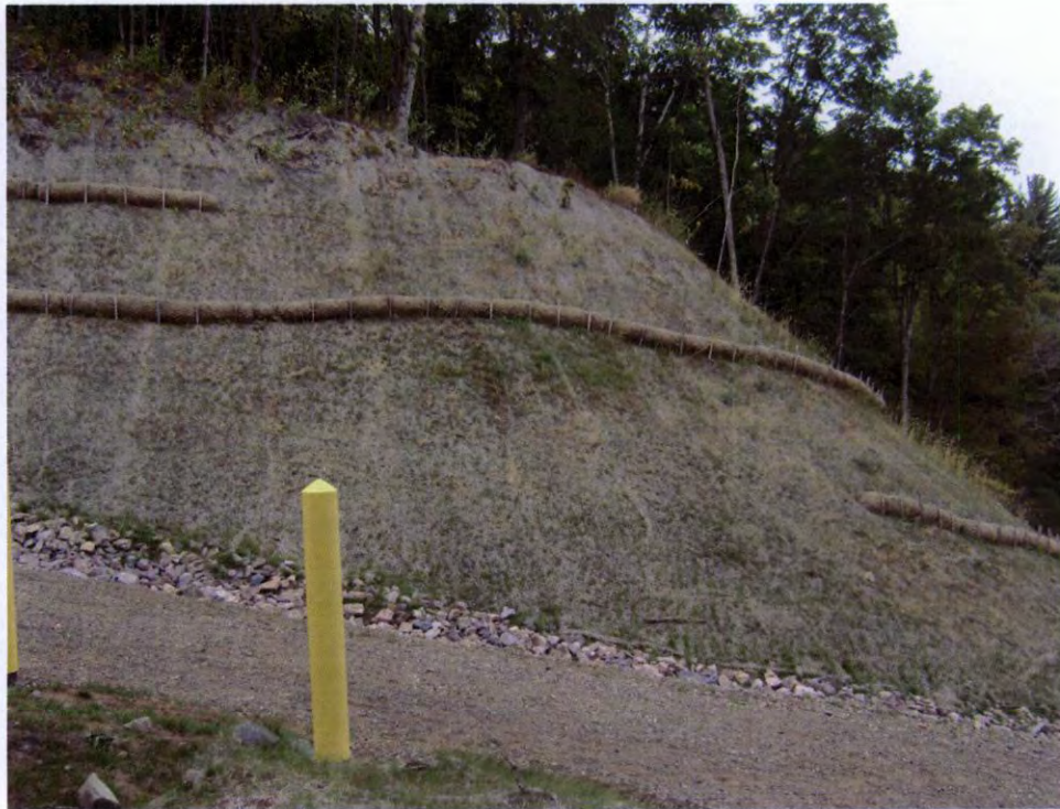
RM-10 looking north (North side of corridor)
