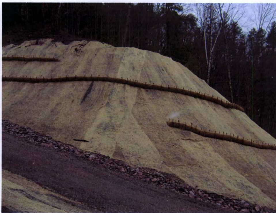
RM-10 looking northwest (North side of corridor)
