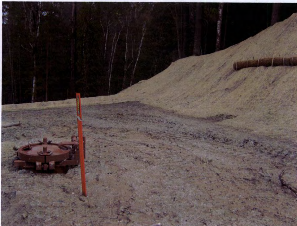
RM-10 looking east (South side of corridor)
