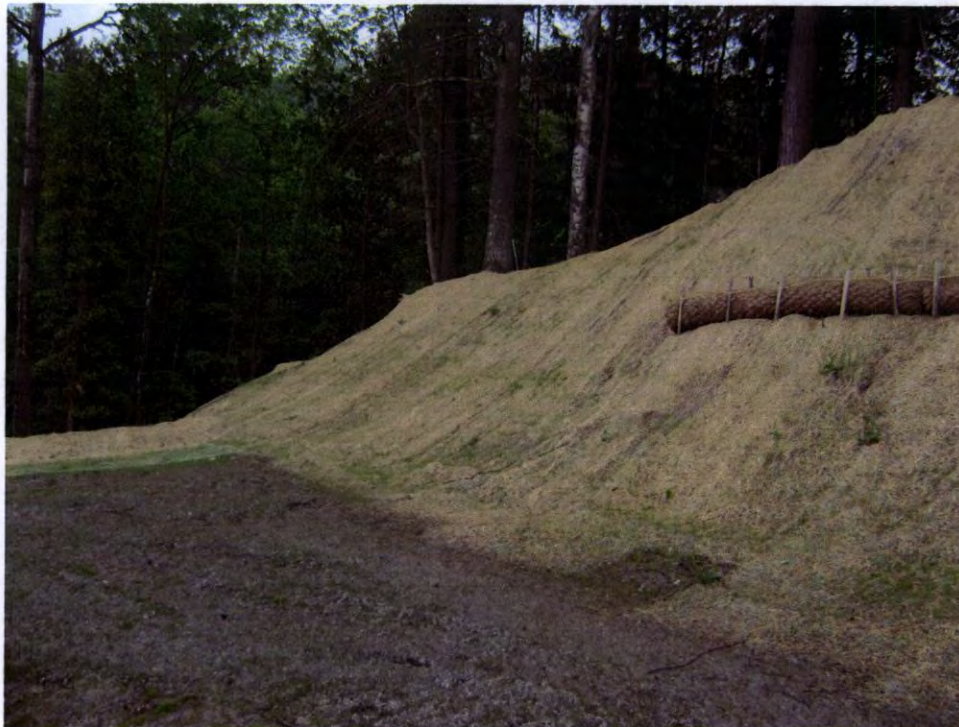
RM-10 looking east (South side of corridor)
