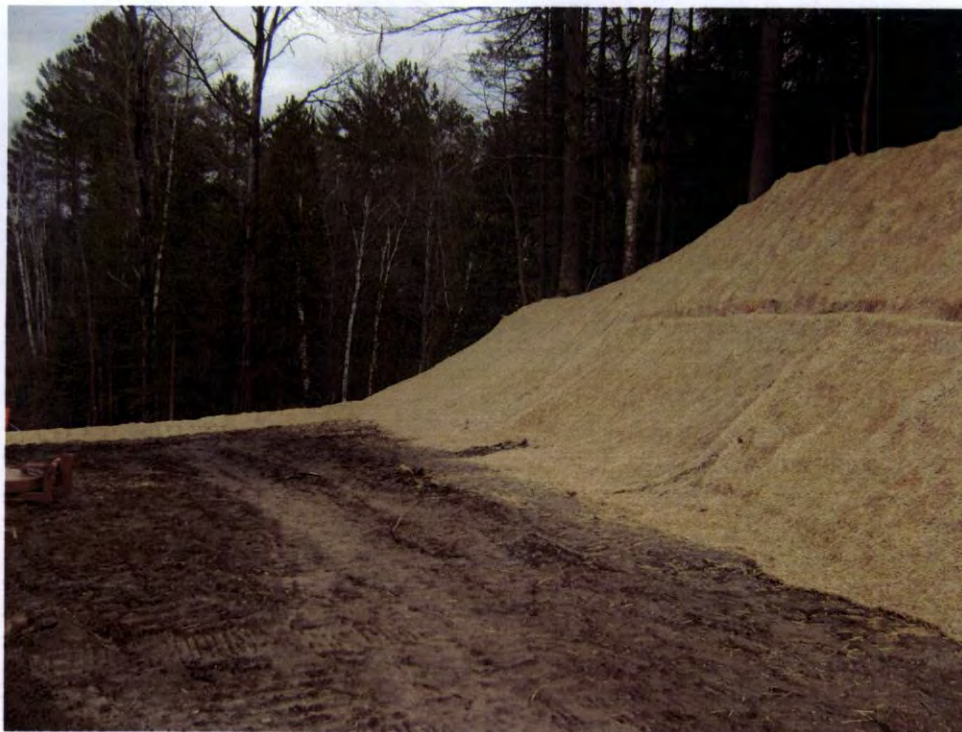
RM-10 looking east (South side of corridor)
