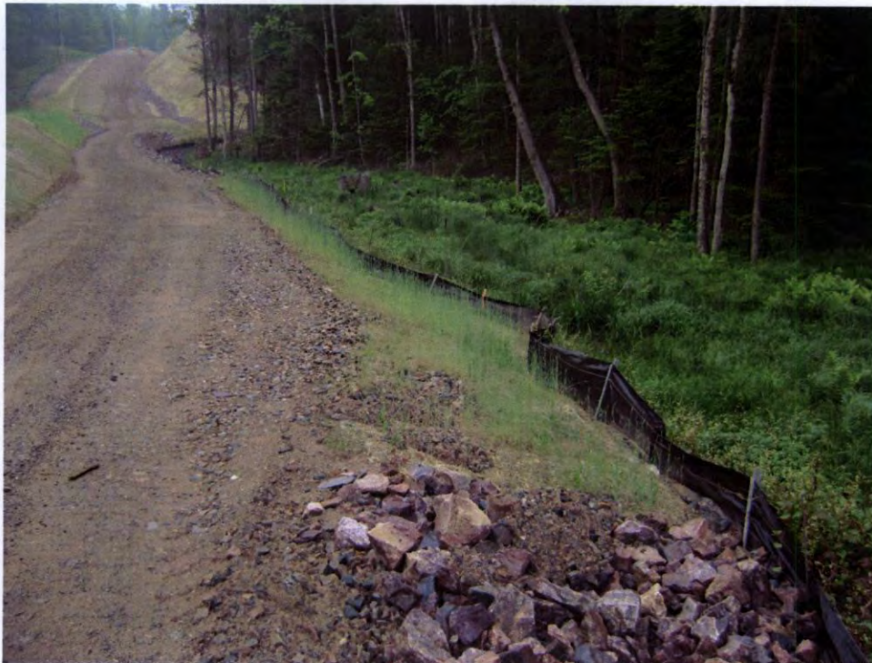
RM-7 looking northeast (South side of corridor)
