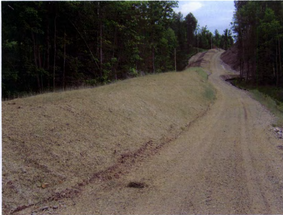
RM-7 looking northeast (North side of corridor)
