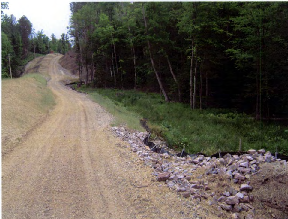
RM-7 looking northeast (South side of corridor)
