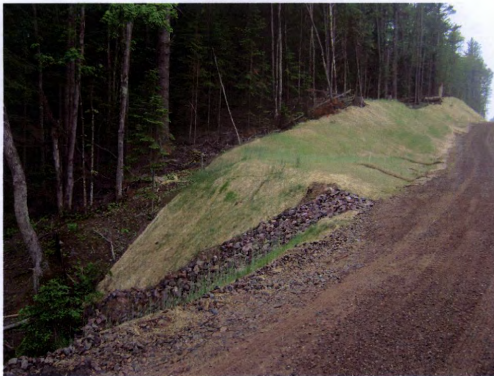
RM-8 looking southwest (South side of corridor)
