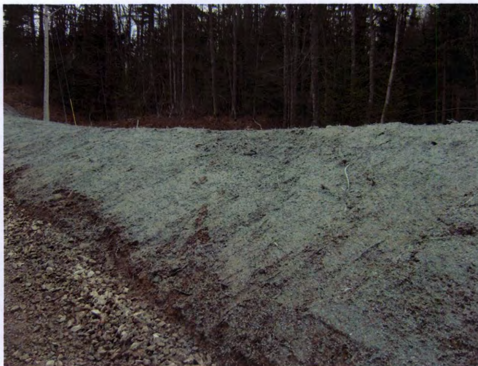
RM-8 looking northwest (North side of corridor)
