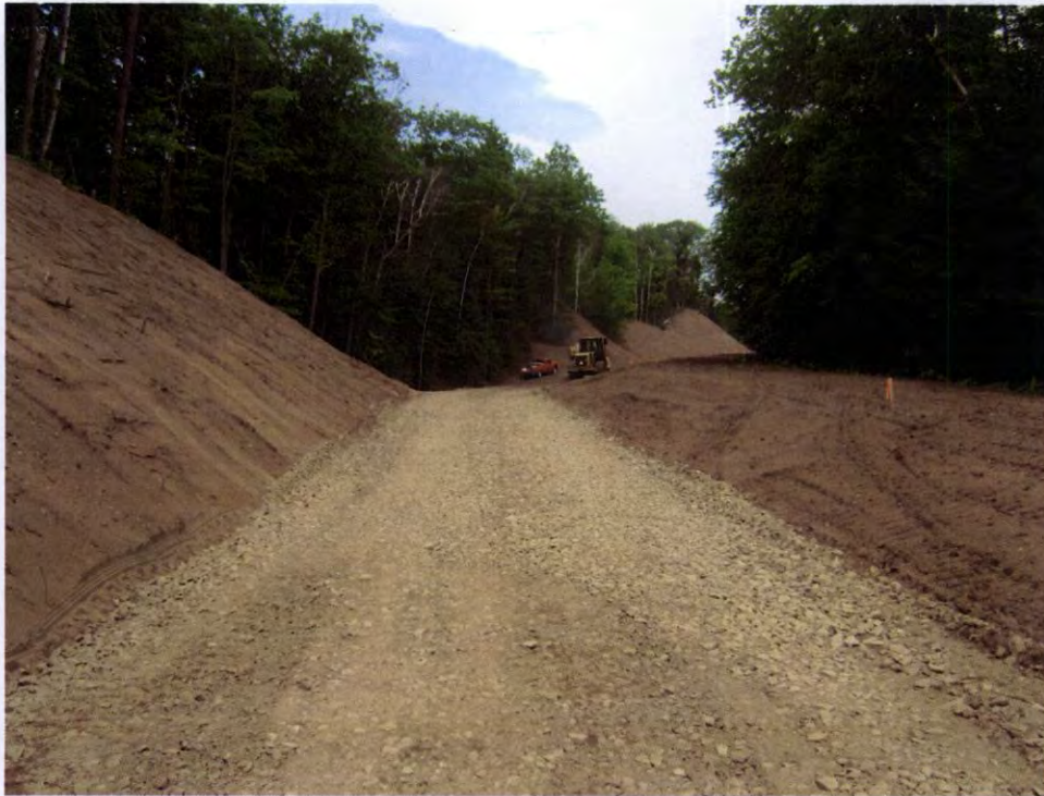
Final grade/topsoil placed between DRM-1 and RM-1
