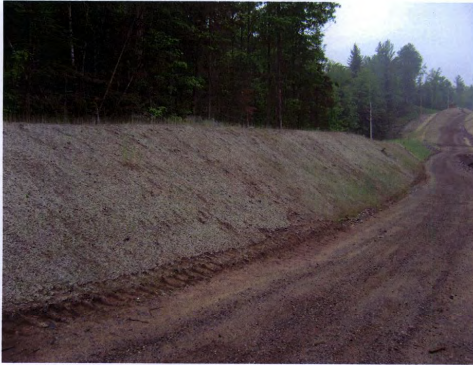
RM-7 looking northeast (North side of corridor)
