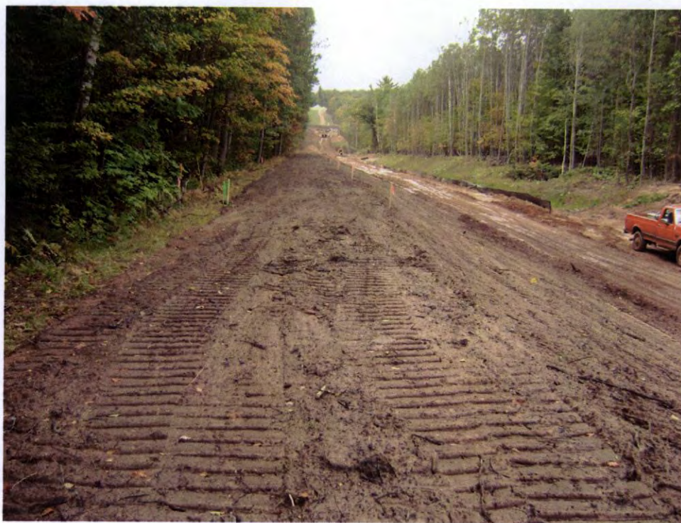
Final Grade/topsoil near RM-4
