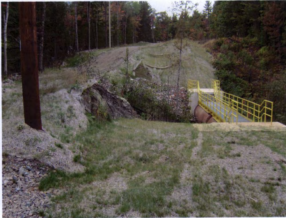
RM-9 looking west (South side of corridor)
