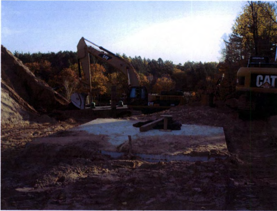
Rough grade being completed near RM-10
