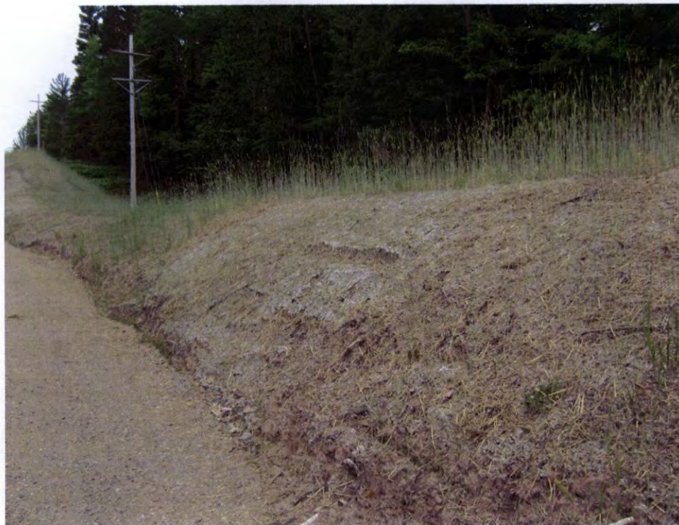
RM-8 looking west (North side of corridor)
