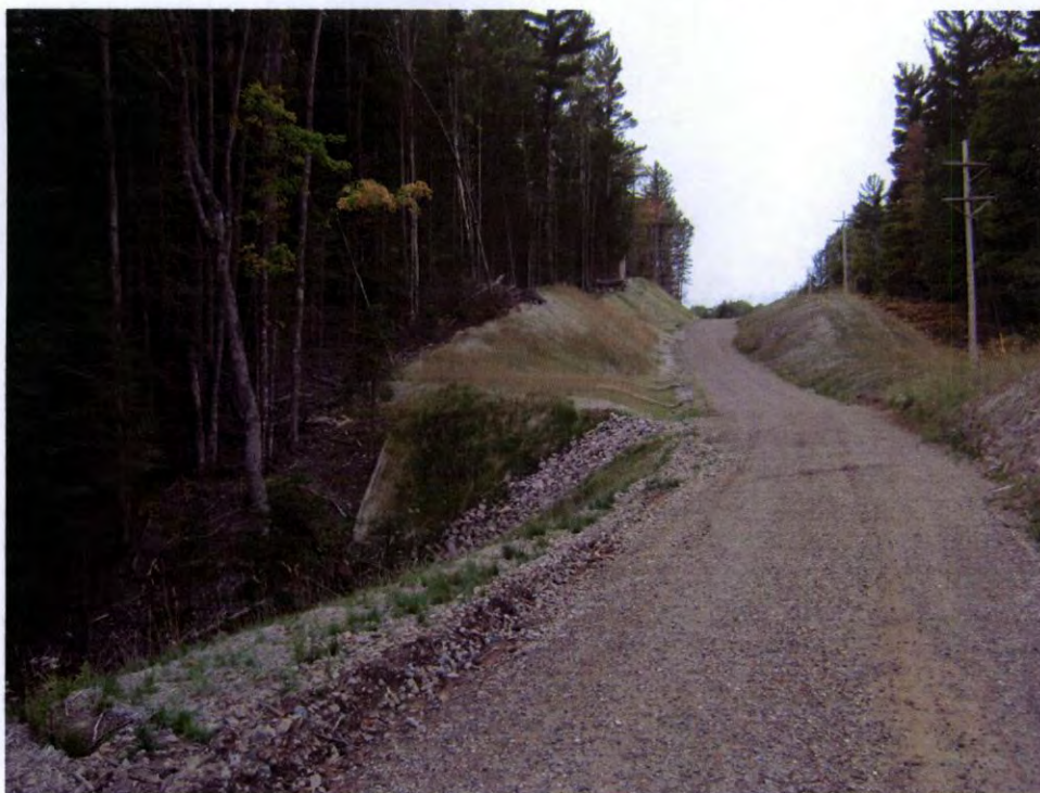
RM-8 looking southwest (South side of corridor)
