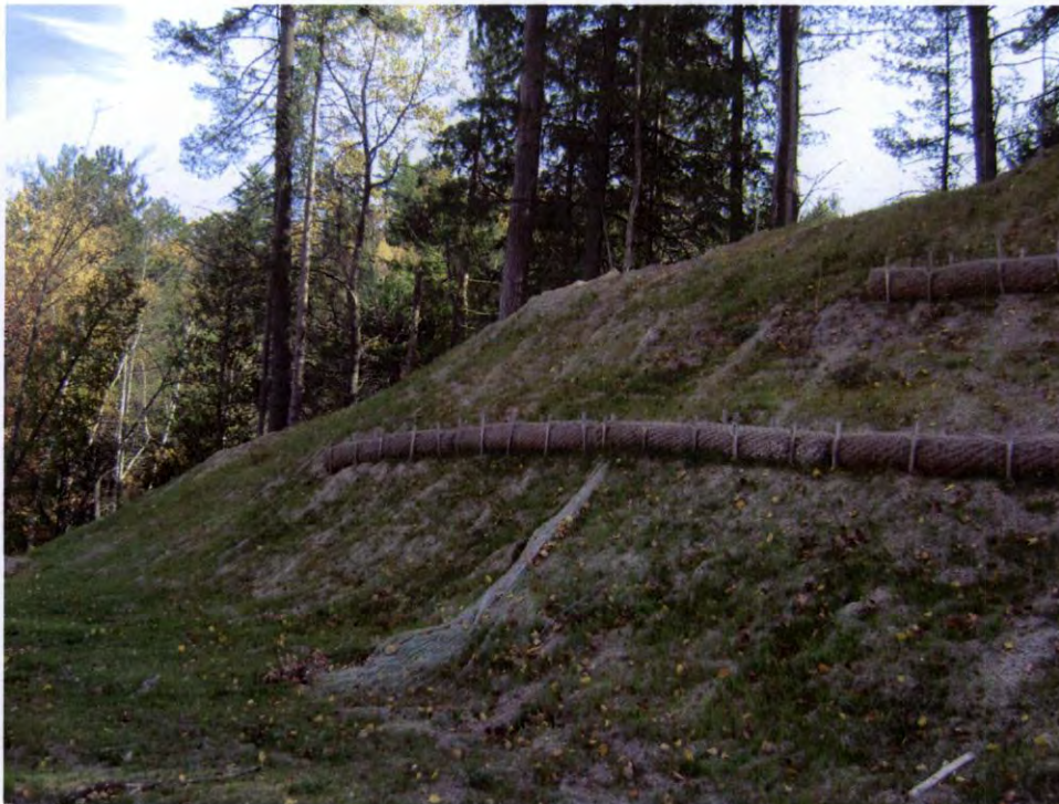
RM-10 looking east (South side of corridor)
