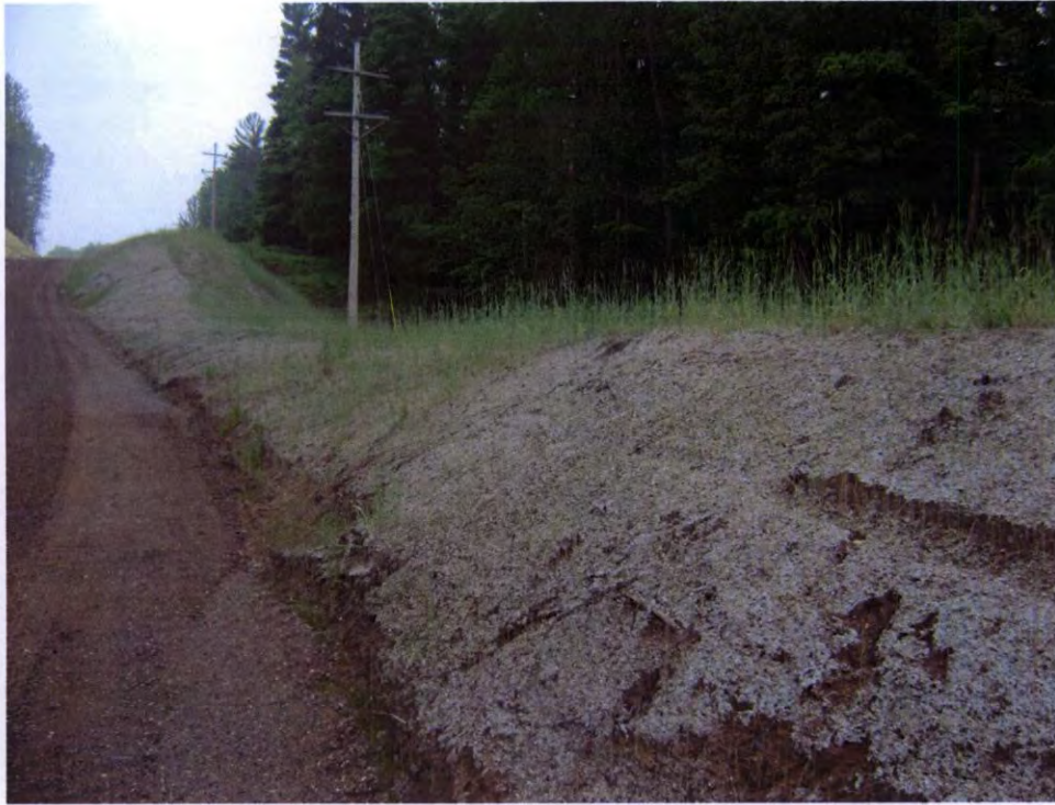
RM-8 looking west (North side of corridor)
