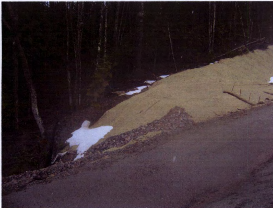
RM-8 looking southwest (South side of corridor)
