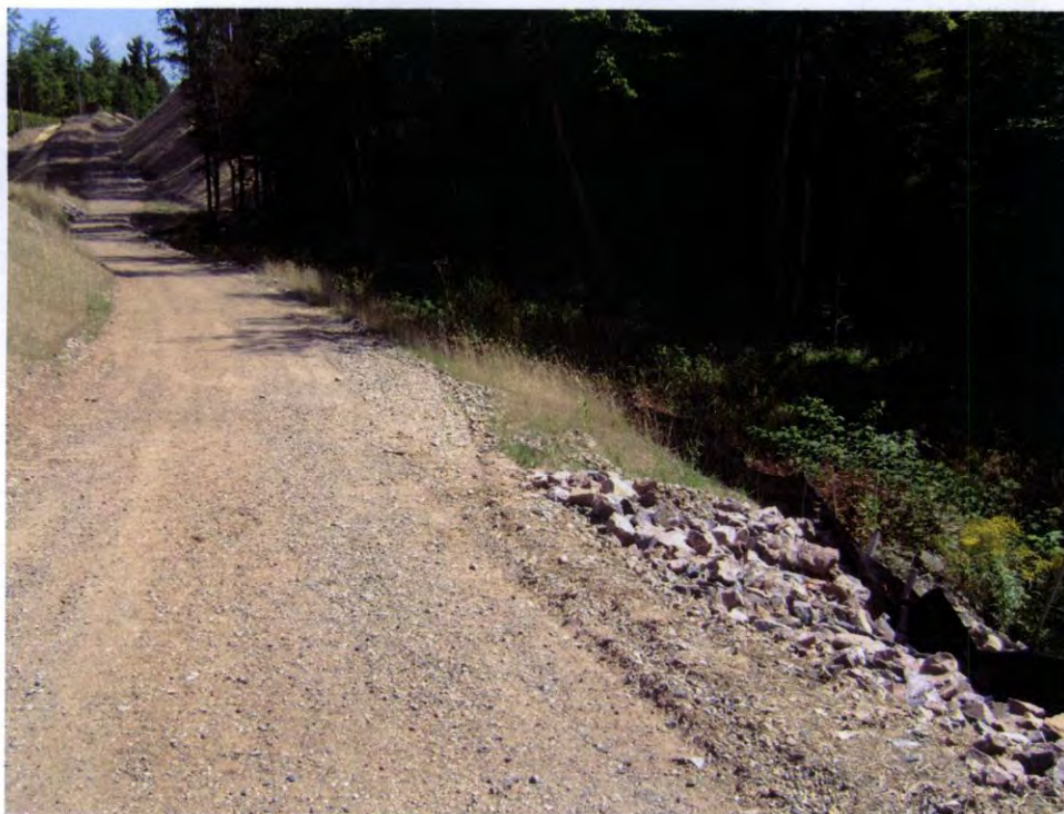
RM-7 looking northeast (South side of corridor)
