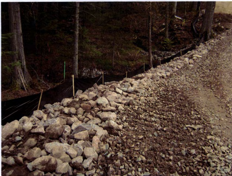
RM-9 looking southwest (South side of corridor)
