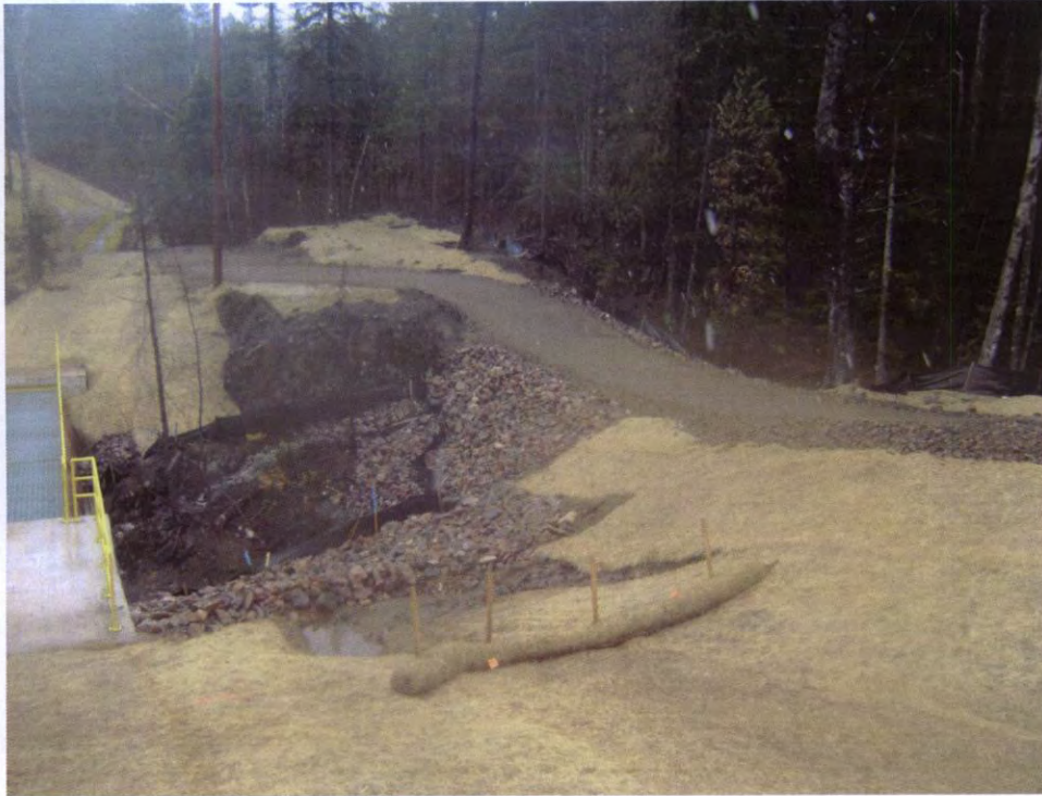
RM-9 looking east (South side of corridor)
