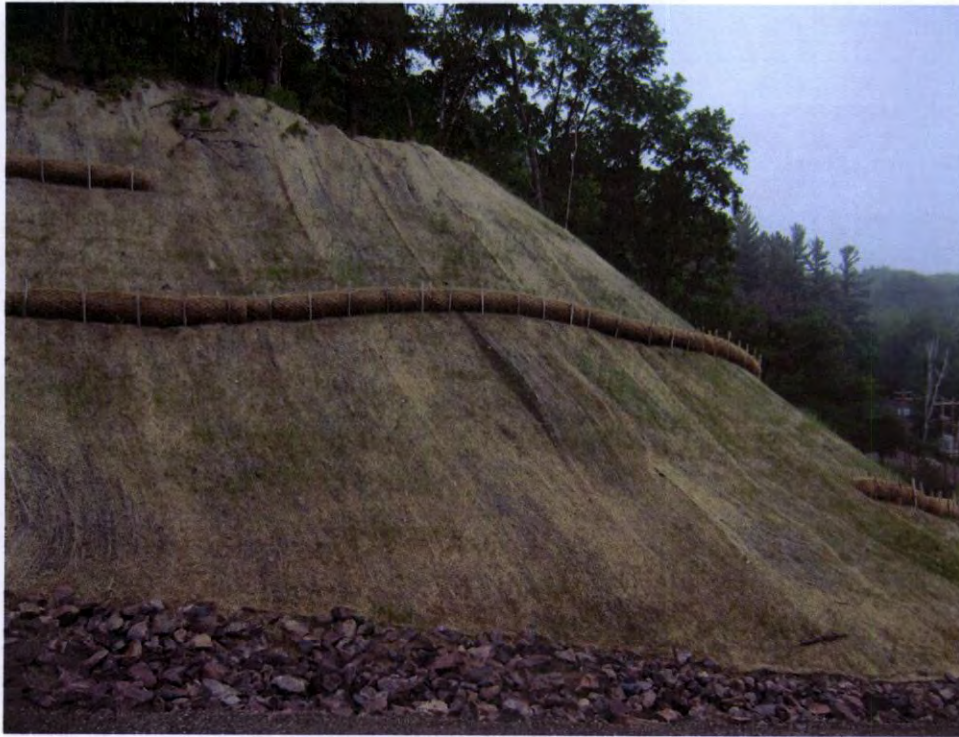
RM-10 looking north (North side of corridor)
