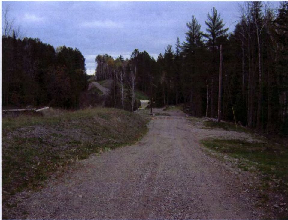
Overall site vegetation between RM-8 and RM-9 (Looking down-stream of penstock flow)
