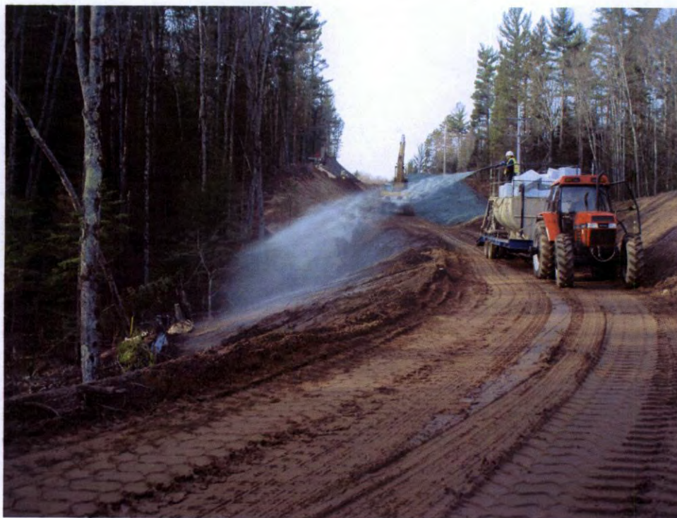
Final grade/topsoil and hydro seeding near RM-8
