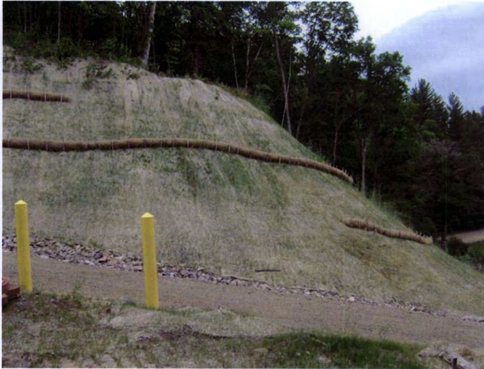
RM-10 looking north (North side of corridor)
