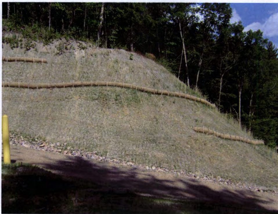
RM-10 looking north (North side of corridor)
