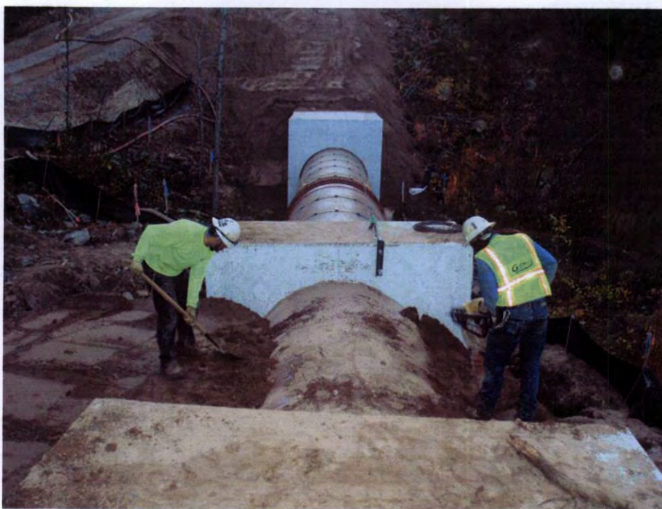
Topsoil placement near RM-9
