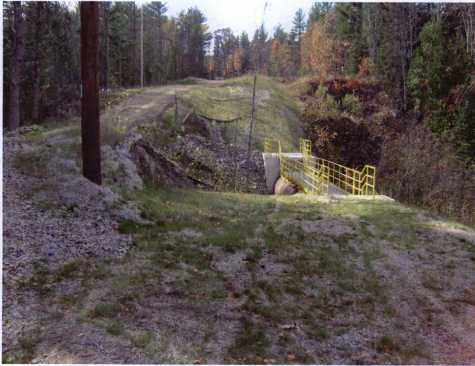
RM-9 looking west (South side of corridor)
