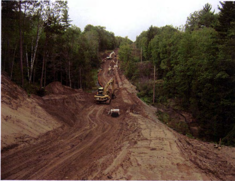
Rough grade being completed near RM-7
