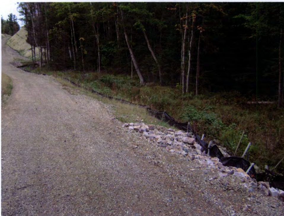
RM-7 looking northeast (South side of corridor)
