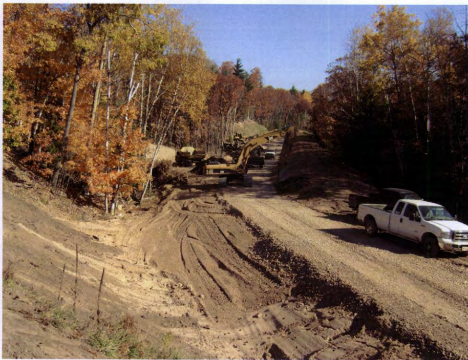
Beginning of topsoil placement near dam embankment
