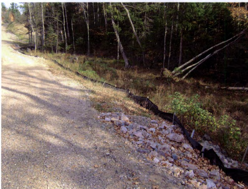
RM-7 looking northeast (South side of corridor)
