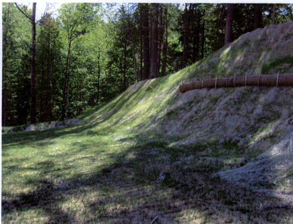
RM-10 looking east (South side of corridor)
