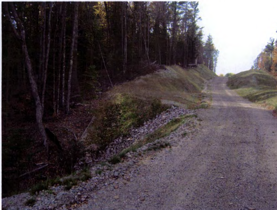
RM-8 looking southwest (South side of corridor)
