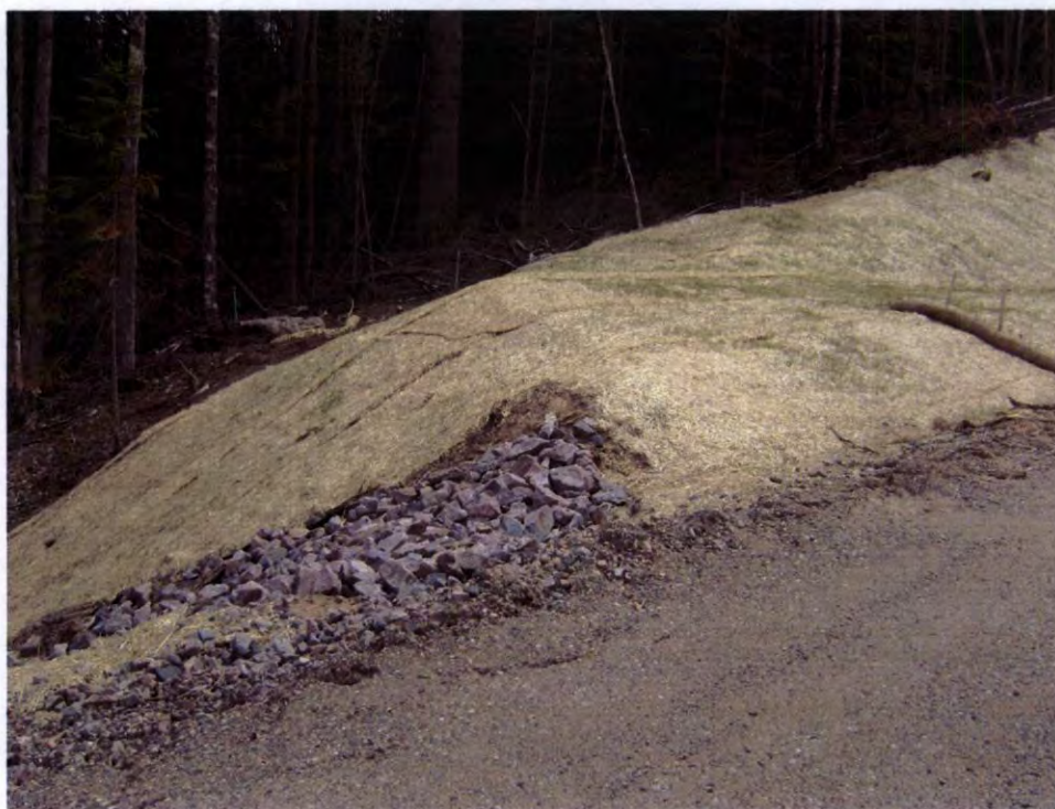
RM-8 looking southwest (South side of corridor)
