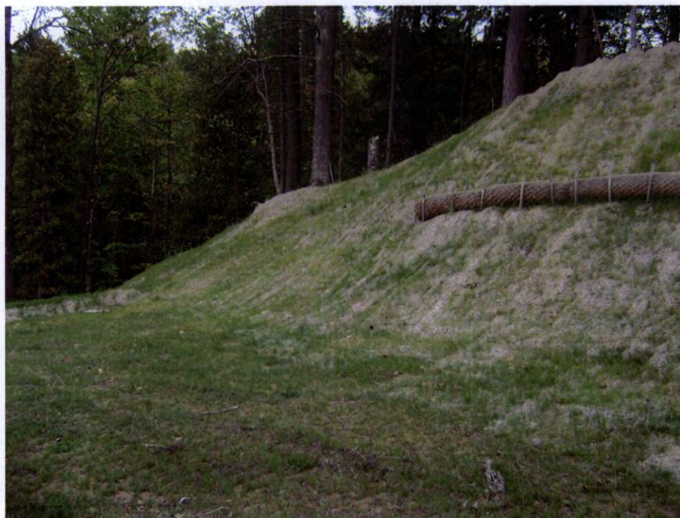
RM-10 looking east (South side of corridor)
