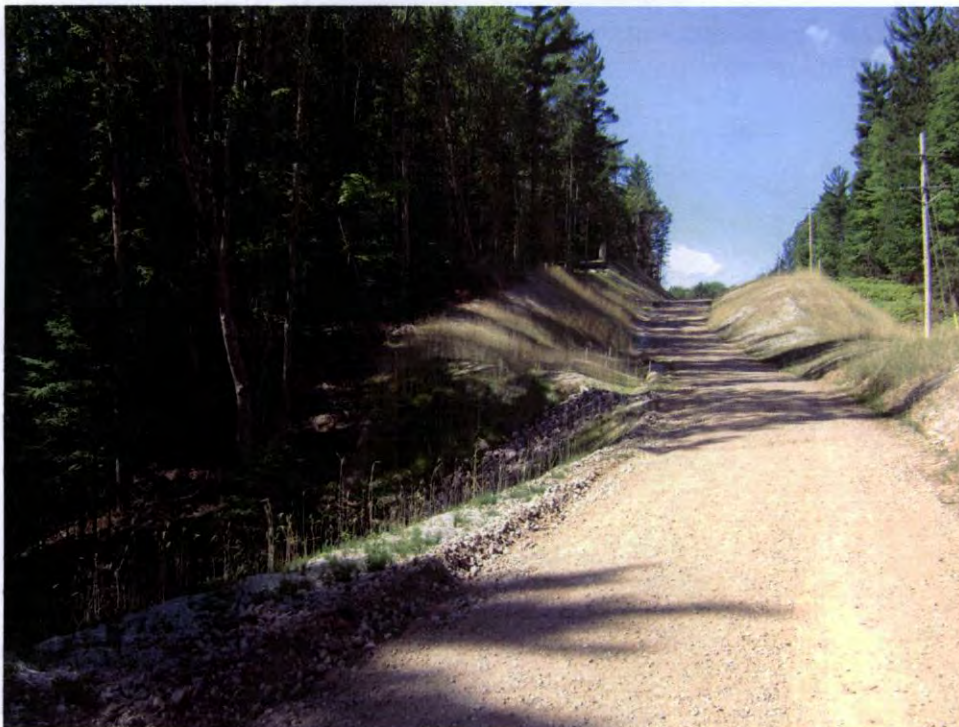
RM-8 looking southwest (South side of corridor)
