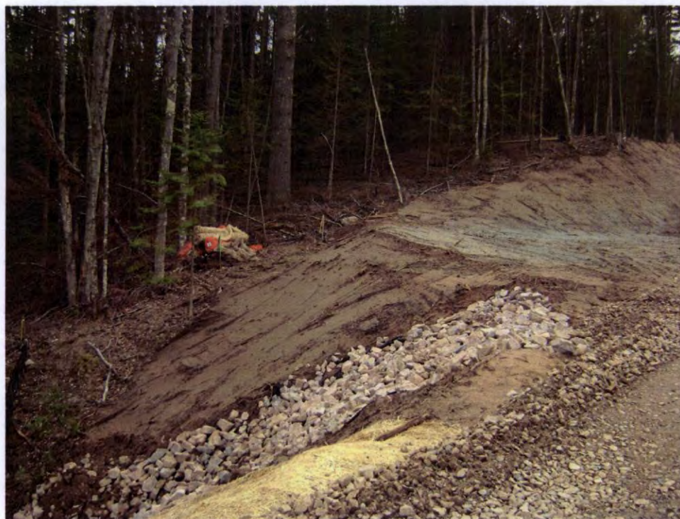
RM-8 looking southwest (South side of corridor)
