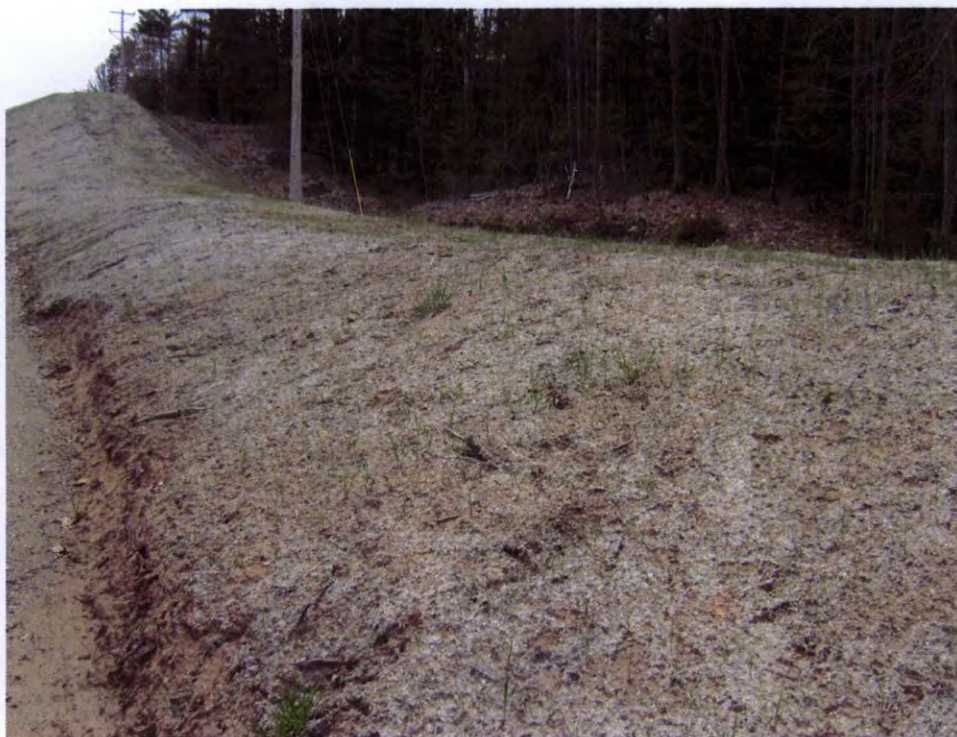
RM-8 looking west (North side of corridor)
