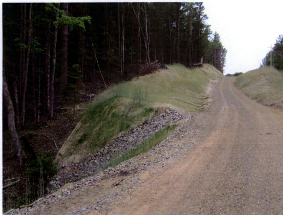
RM-8 looking southwest (South side of corridor)
