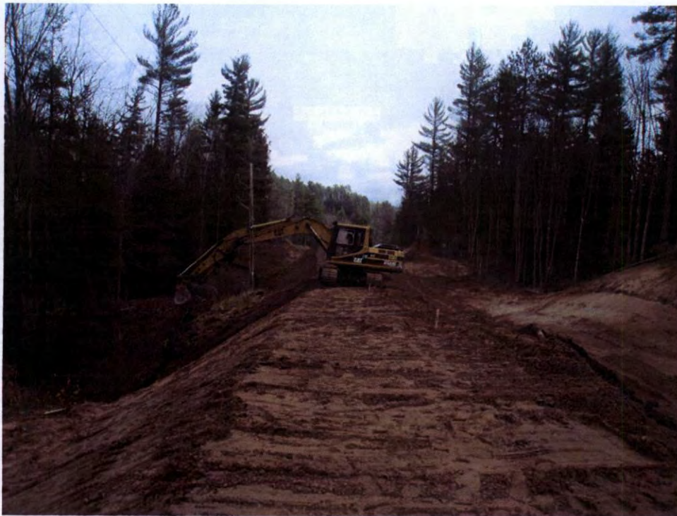
Topsoil placement between RM-7 and RM-8
