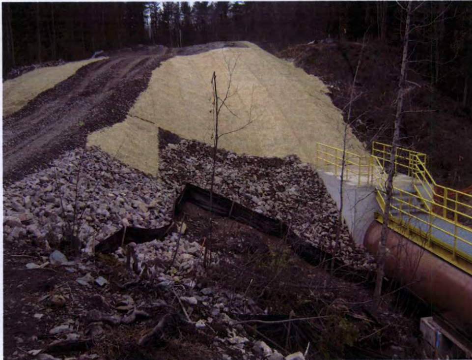
RM-9 looking west (North side of corridor)
