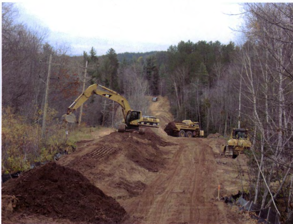
Topsoil placement near RM-6
