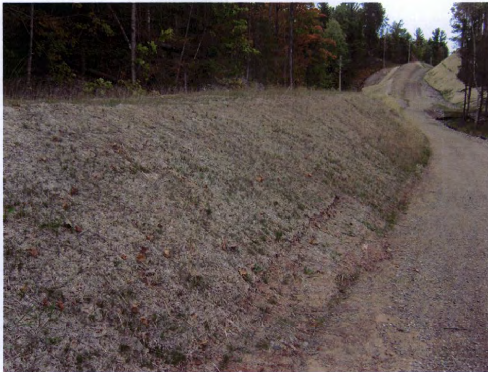
RM-7 looking northeast (North side of corridor)
