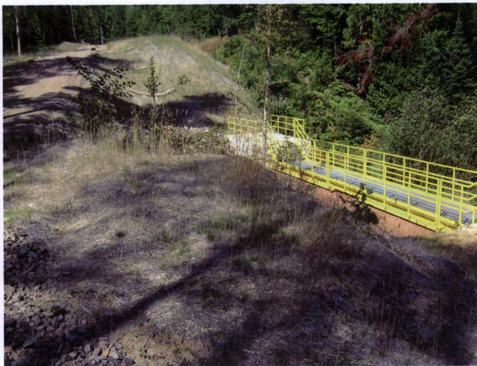
RM-9 looking northwest (South side of corridor)
