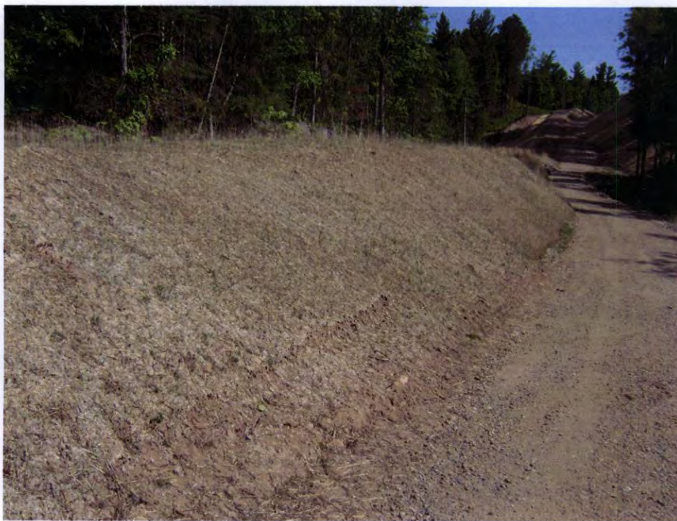
RM-7 looking northeast (North side of corridor)
