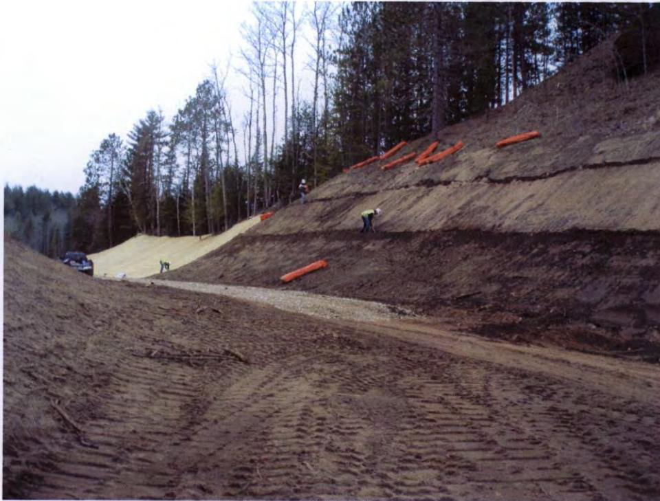
Installation of mulch blanket near RM-10
