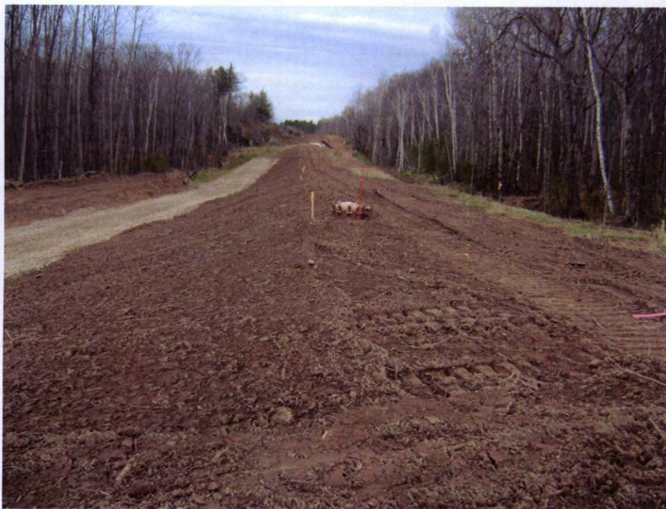
Final grade/topsoil near RM-5
