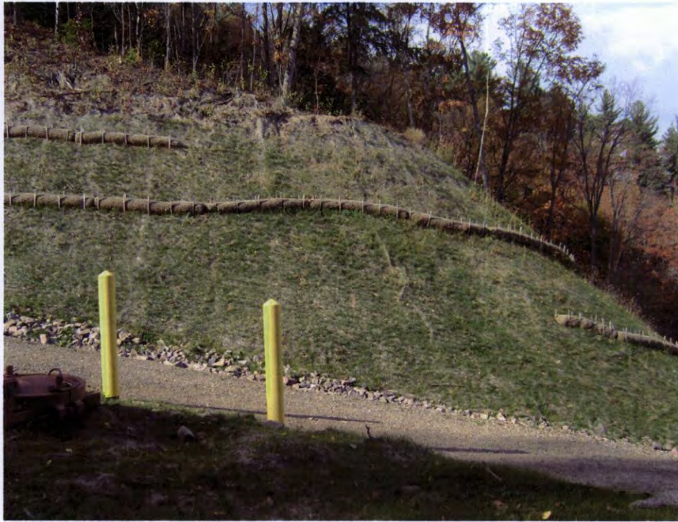
RM-10 looking north (North side of corridor)
