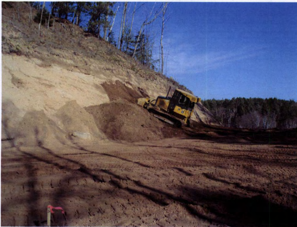
Topsoil placement near RM-10
