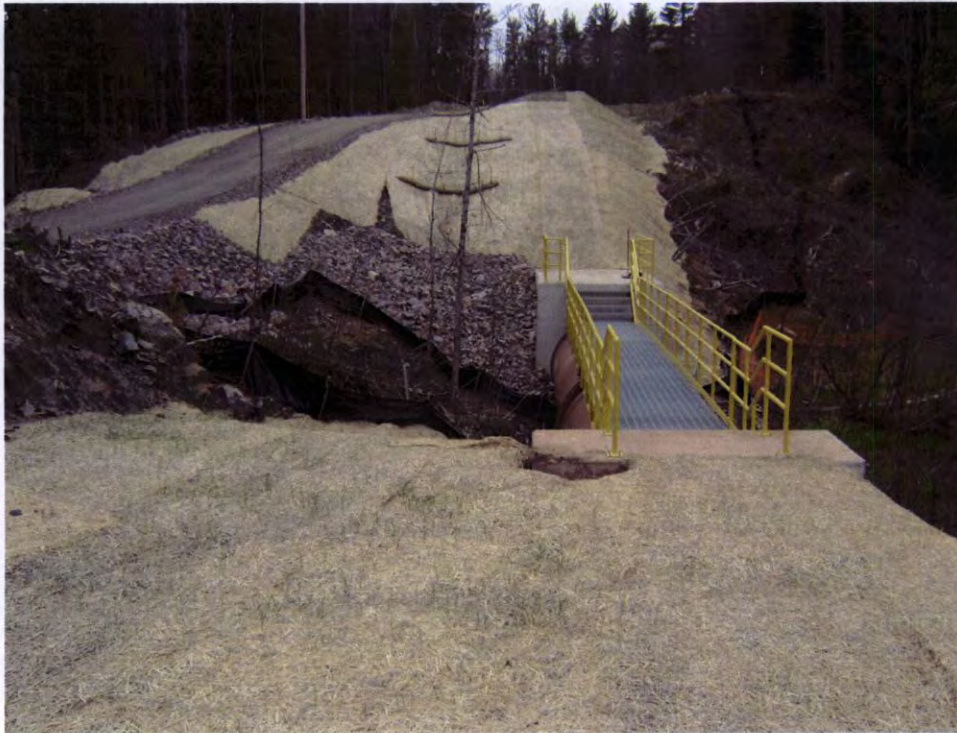
RM-9 looking west (South side of corridor)
