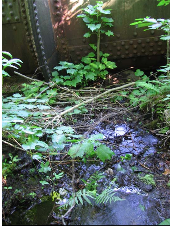
Photo 23. Stream #4 flowing beneath the penstock.
