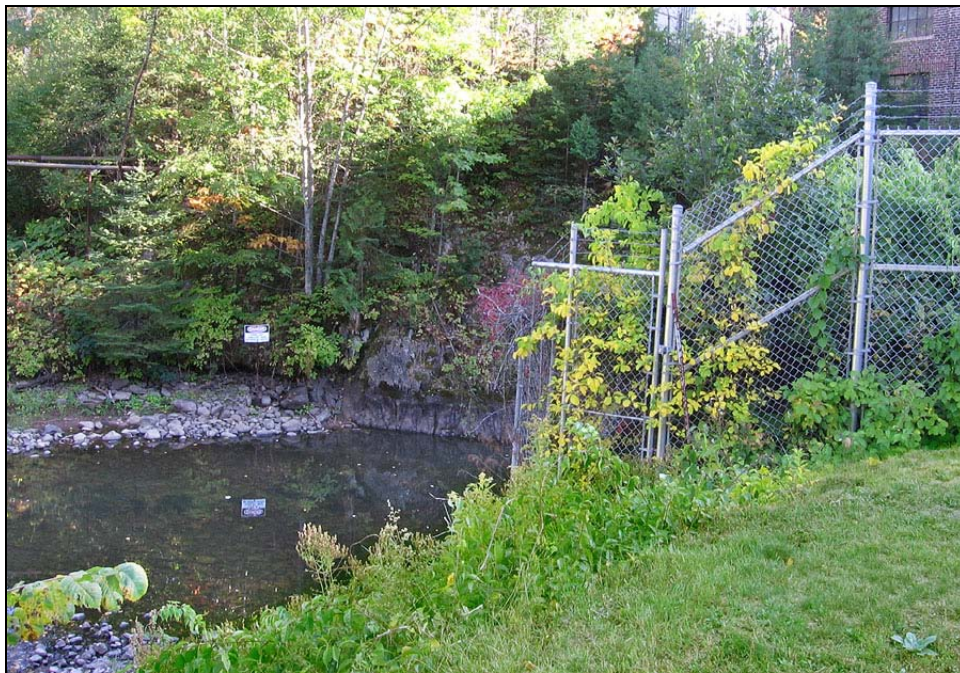
Photo 16. Stream #1, outflow from the penstock and powerhouse.
