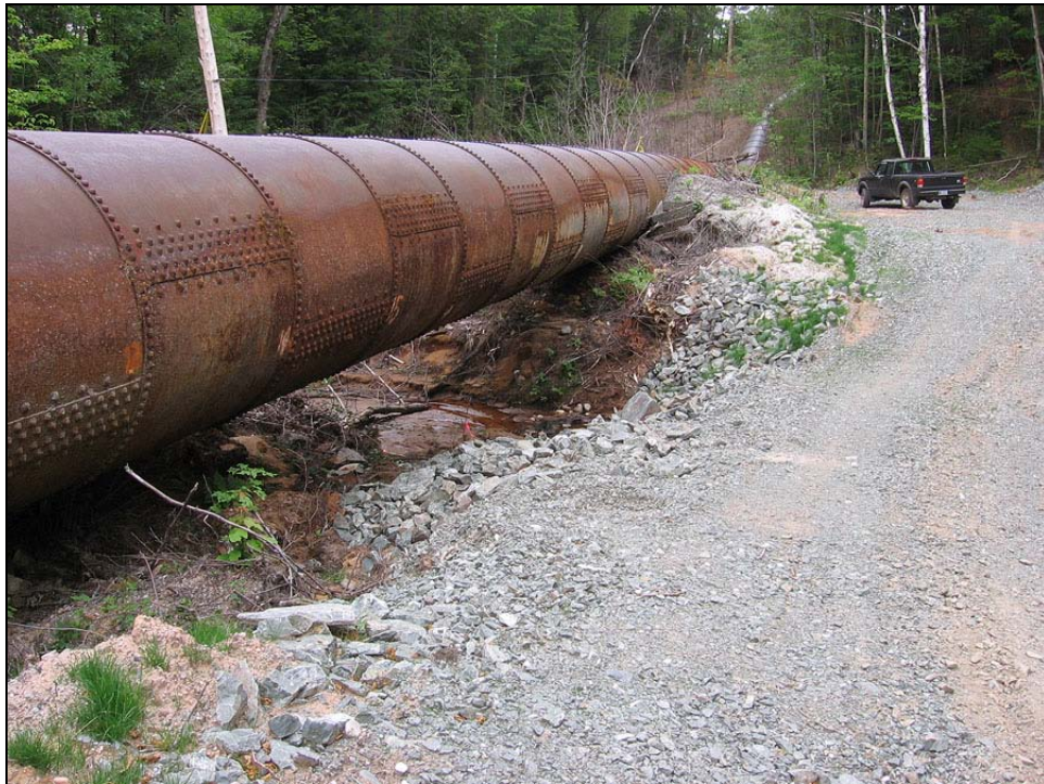
Photo 28. Stream #6 flowing beneath the access road and penstock.
