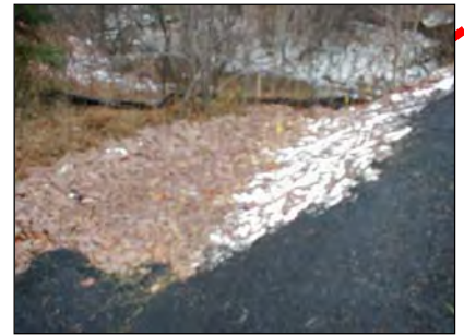
Site #8 - CR 510, Midway Creek (after). Elimination of sand berm. Road was paved and storm water rerouted into the re-sloped ditch with a water diversion at the end to dissipate the flow of runoff.
