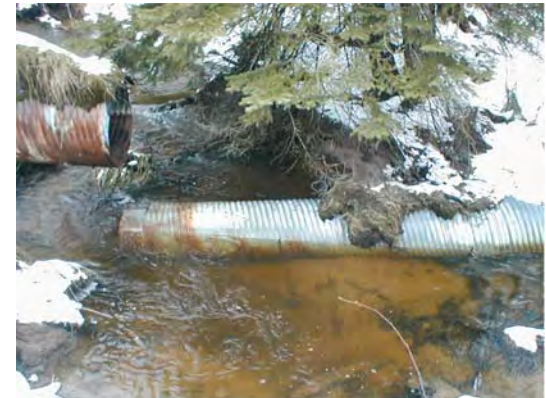
Culvert on Brickyard Creek
