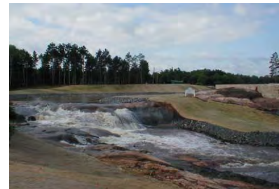
Rip-rap and newly seeded grass help prevent erosion
