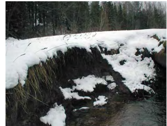
Scouring of stream bank along Brickyard Creek
