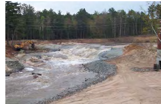
Tourist Park dam gave way under pressure from floodwaters
