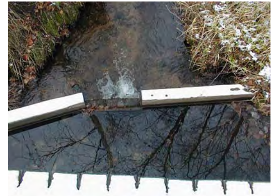
Small residential dam along Brickyard Creek
