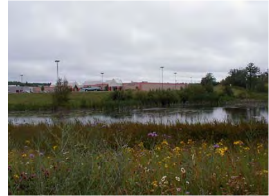
A detention basin retains and treats stormwater
