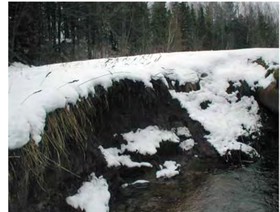
Erosion along Brickyard Creek
