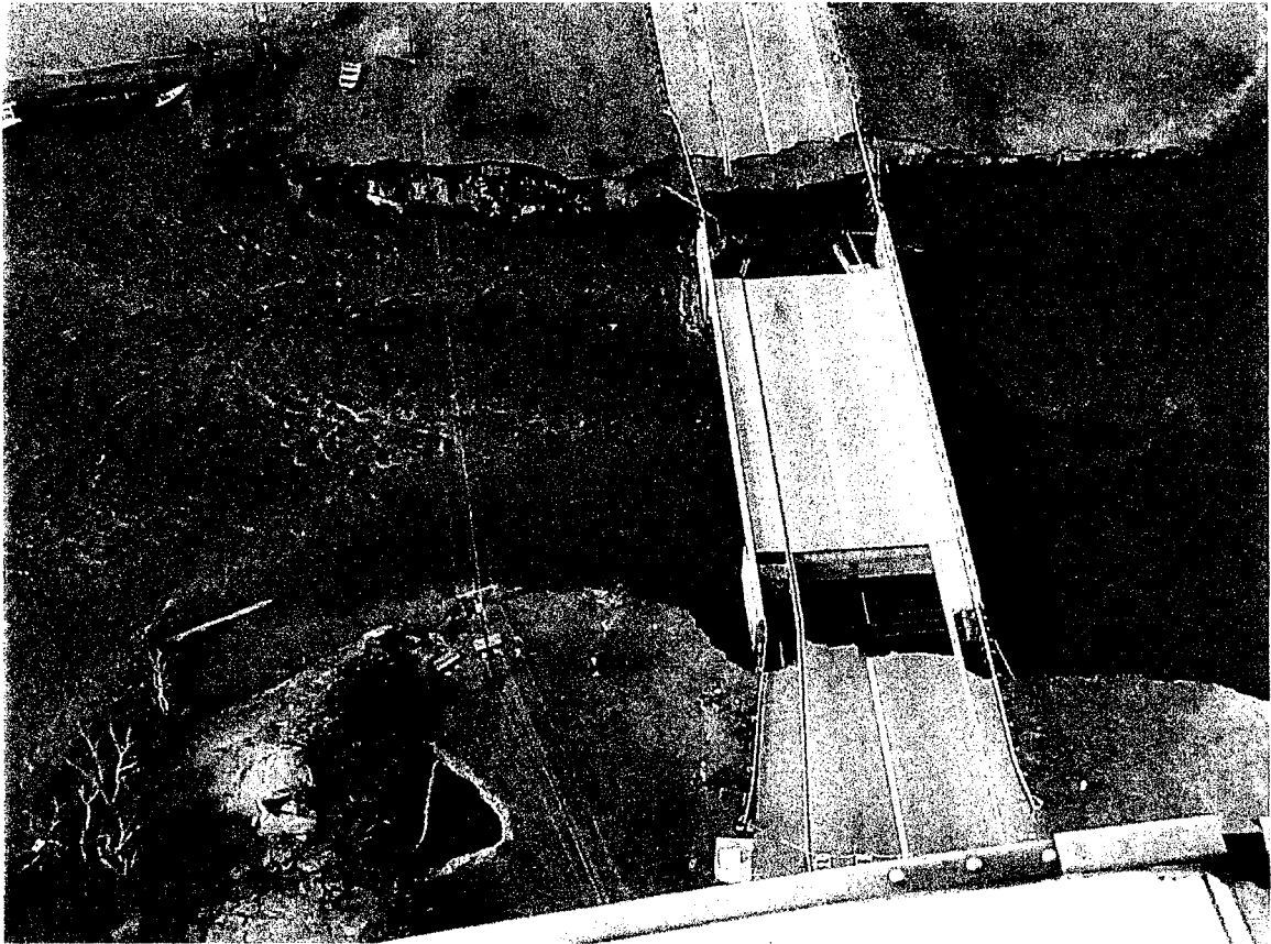
Figure 3.6.5-1 Bridge at mouth of Dead River after fuse plug breach
