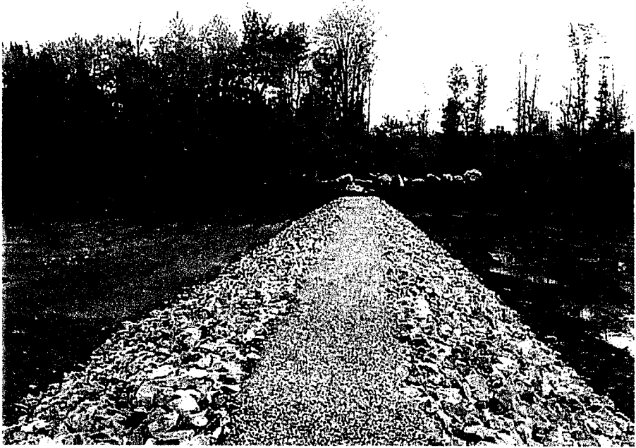
Fuse plug embankment at end of construction, October 8, 2002
