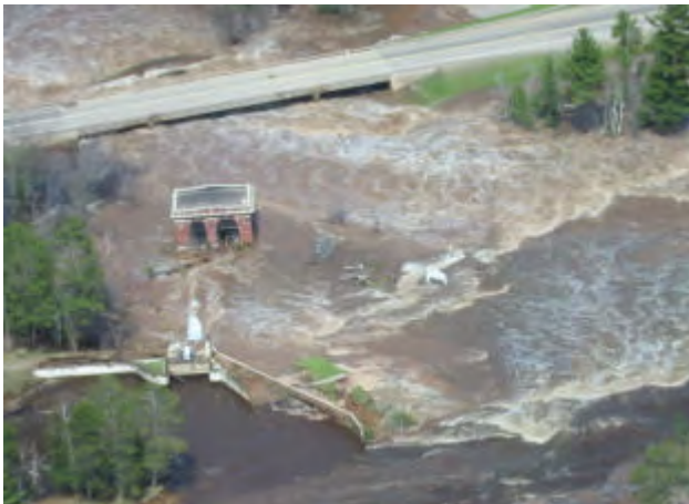
Photo 13. Tourist Park dam breach. Source MDNR 5/15/03
