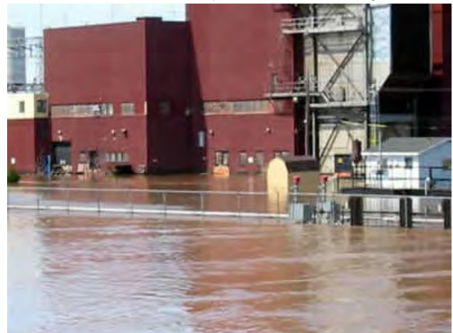
Photo 16. Flooded Presque Isle Power Plant 5/15/03. Source: Marquette County
