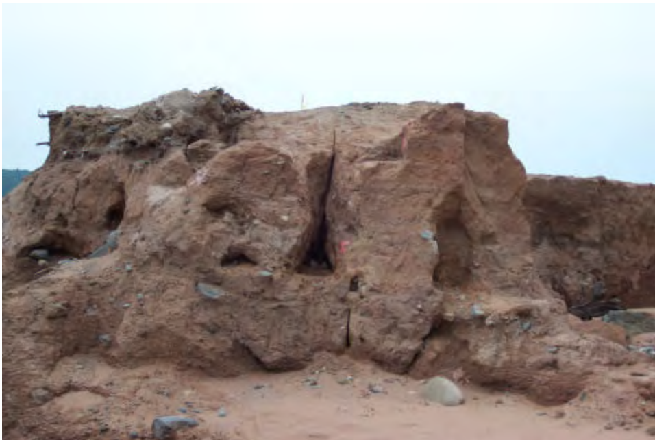
Figure 6 View of similar erosional features as described in Figure 5. Note the association of a vertical fracture with two of these erosional pockets. View is of an “island” remnant downstream of former fuse plug.
