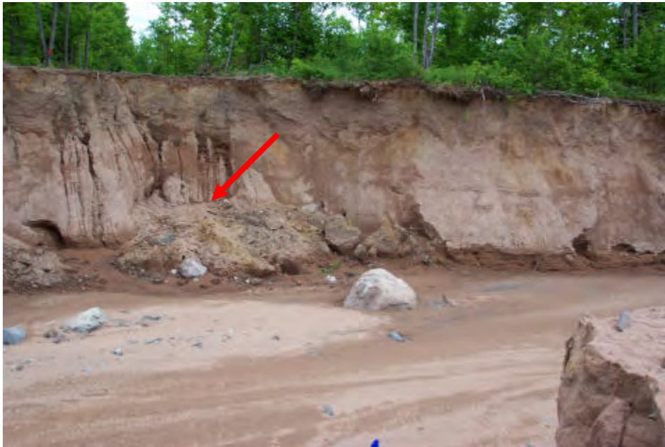
Figure 4 The upper SP-SM unit appears to contain a weak soil structure (weak carbonate cementation?) that when disturbed loses strength and crumbles (pile at arrow). This unit has a low dry strength and is easily broken by light finger pressure. View is of left channel downstream of former fuse plug.
