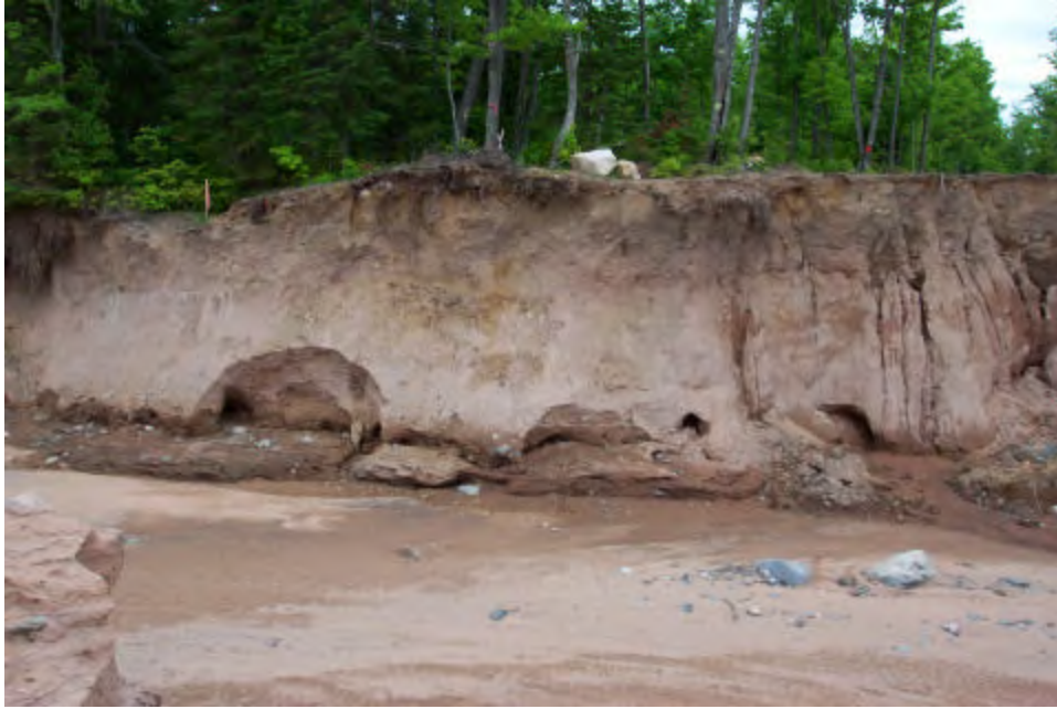
Figure 3 Overall view of "Coarse-textured glacial till." Note vertical erosional gullies (at right) and circular erosional features near base. Upper horizon is oxidized and contains some roots from surface vegetation. This deposit stands vertically similar to loess. On surface exposures, this material is dry. This unit likely contains weak carbonate cementation, but is a cohesionless soil. View is of left channel downstream of former fuse plug.
