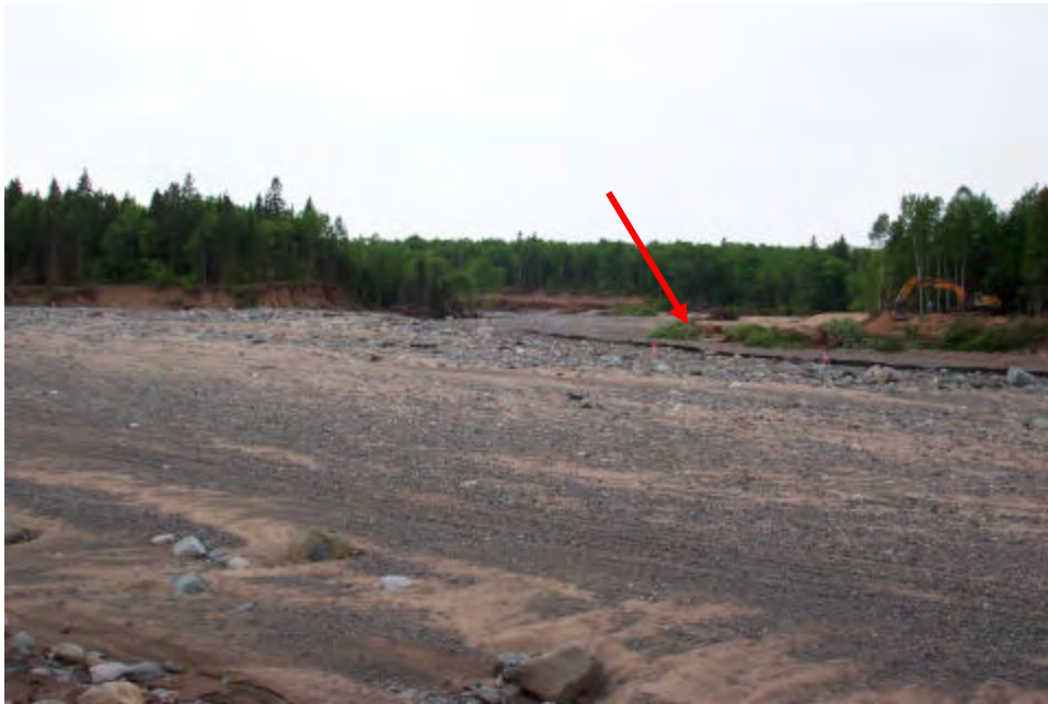
Figure 10 View of channel erosion and flood deposition downstream of former fuse plug. Note the light-colored deposits in the upper right of the photograph (arrow). This shows large amounts of well graded sand that were deposited along an inner bend of the channel alignment, approximately 1,100 feet downstream of the former fuse plug.
