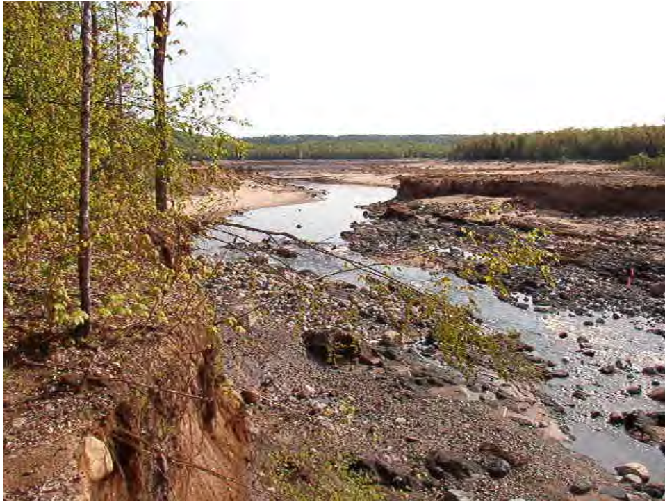
Photograph 3. Silver Lake channel entrance as viewed from the right abutment near Station 0+35. Photograph taken on June 3, 2003.
