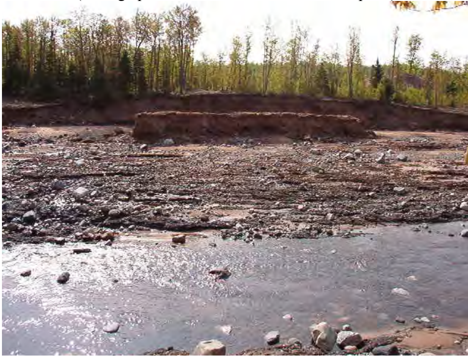
Photograph 5. The left abutment at Station 0+35 where the fuseplug dike was located. According to the STS survey, the top of the remnant section is at elevation 1481 feet. Photograph taken on June 3, 2003.
