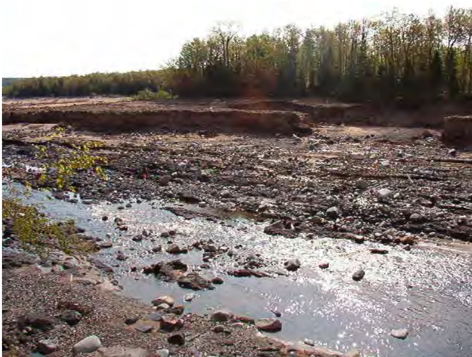
Photograph 4. View of the upstream portion of the channel as viewed from the right abutment near Station 0+35. Photograph taken on June 3, 2003.
