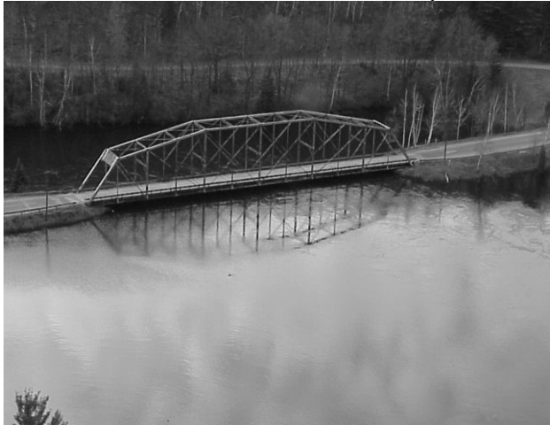
CR 510 Steel Bridge
