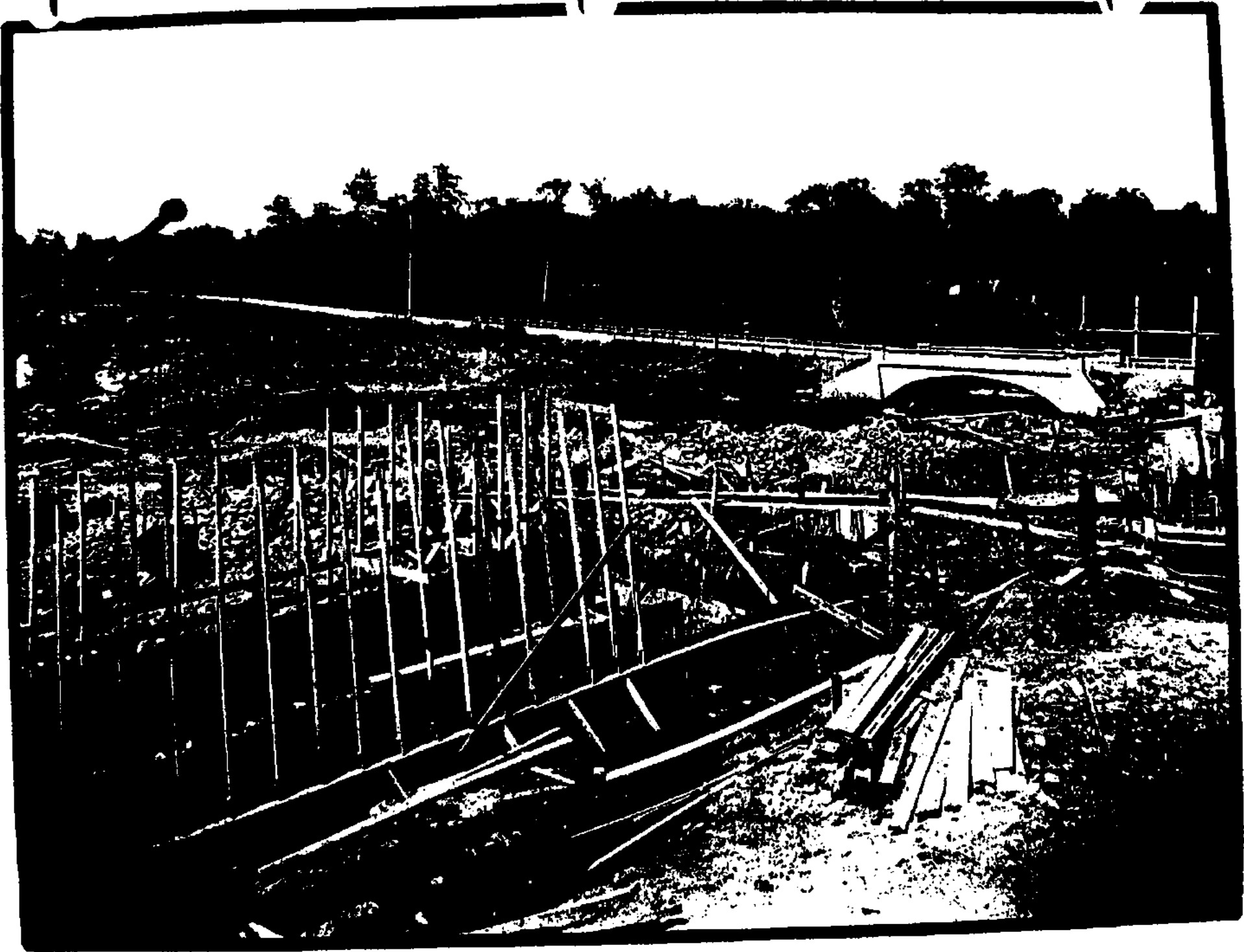
AT TRAIL RIVER WATER POWER PLANT VIEW SHOWING SPILLWAY ERECTING, LOOKING SOUTHWEST
