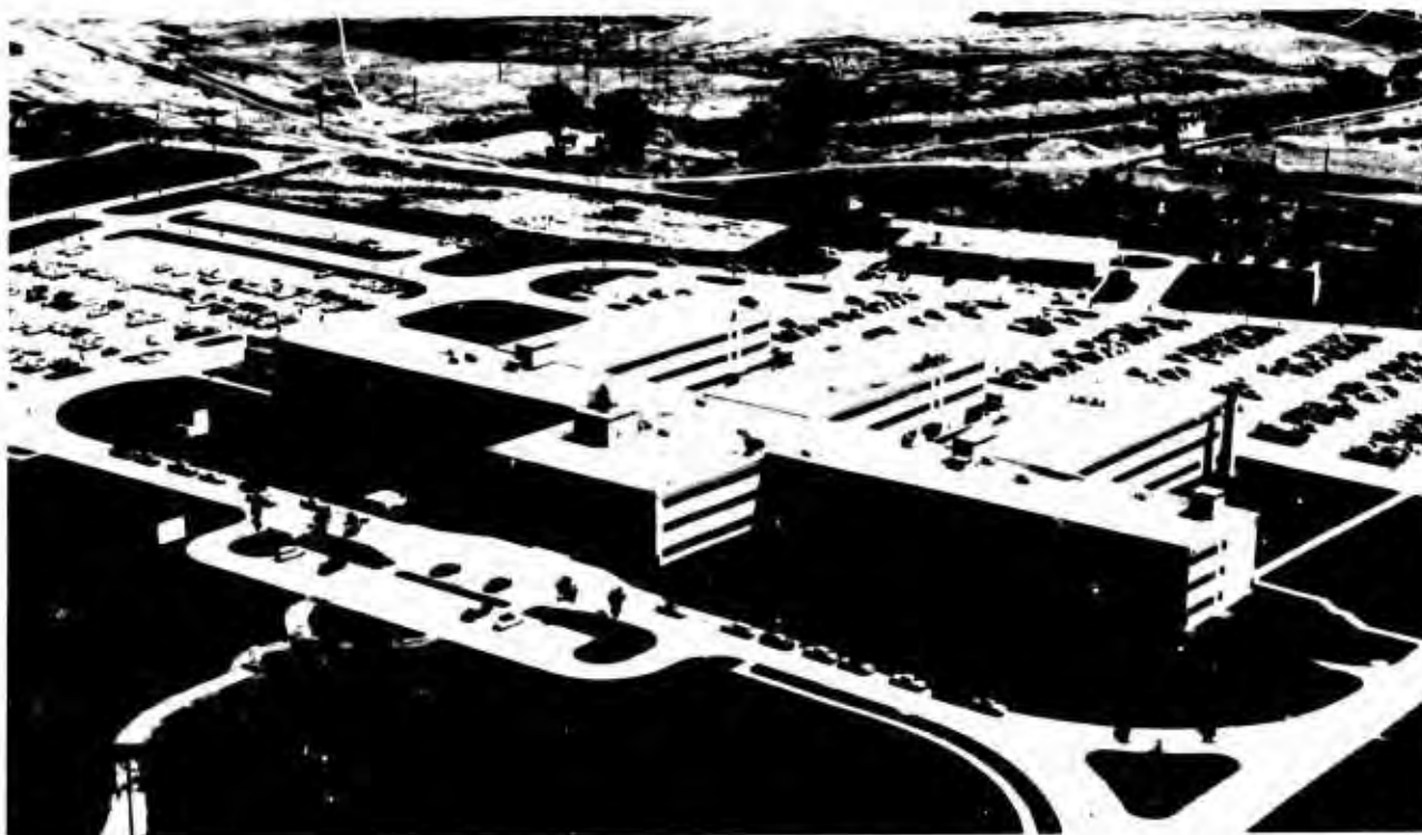
New Headquarters SAC Building, Offutt AFB, Nebraska, 1957
