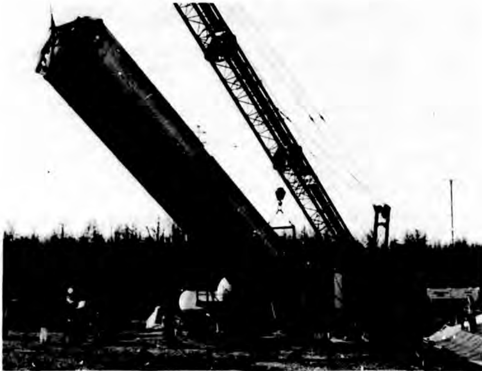
Titan II after removal from silo
