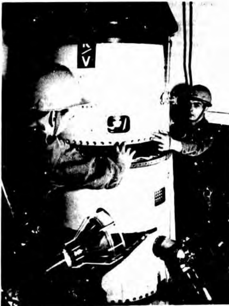
Minuteman II assembly in silo, Grand Forks AFB
