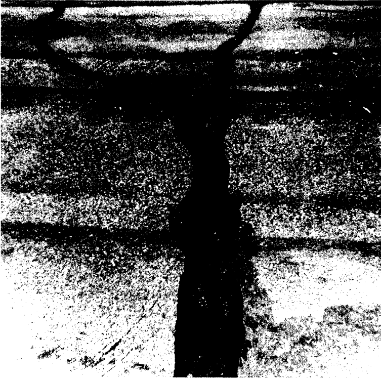
Photo 5. Cracks in taxiway B (feature T14B)
