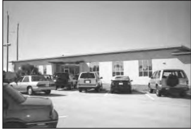
Figure 15. Exterior of Building 1638.
