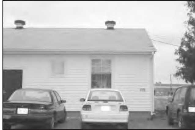
Figure 38. Building 2159 contains all post archaeological collections.
