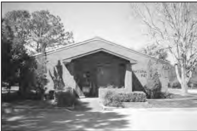
Figure 30. Front entrance of the Natural Resources building.
