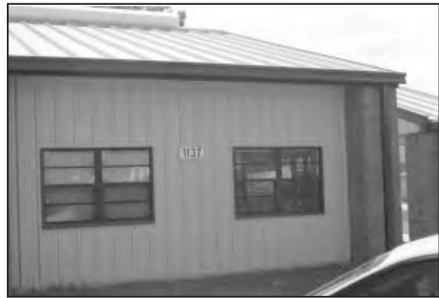
Figure 33. Exterior of Building 1137 where artifacts are stored.
