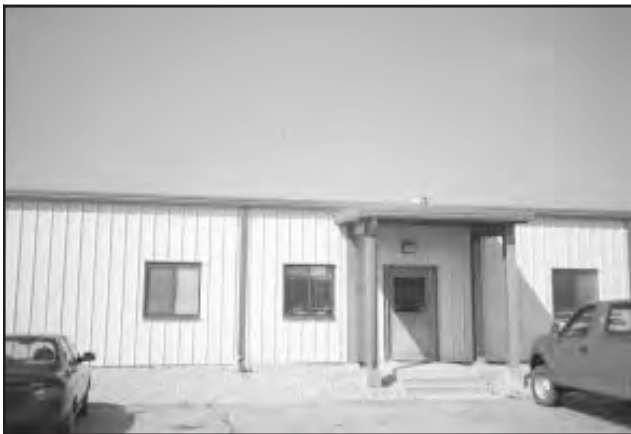
Figure 4. View of Building 1453 showing roof and facade.
