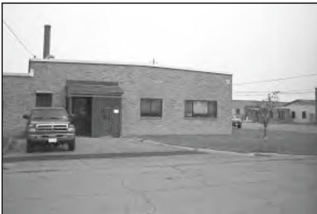
Figure 55. Building 123 contains all of the post's archaeological collections.
