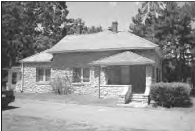
Figure 44. The old pump house now serves as the archaeological collections repository.
