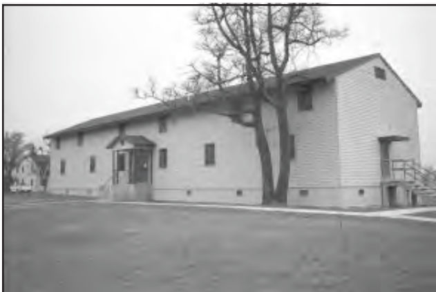
Figure 10. The front of Building 1313.
