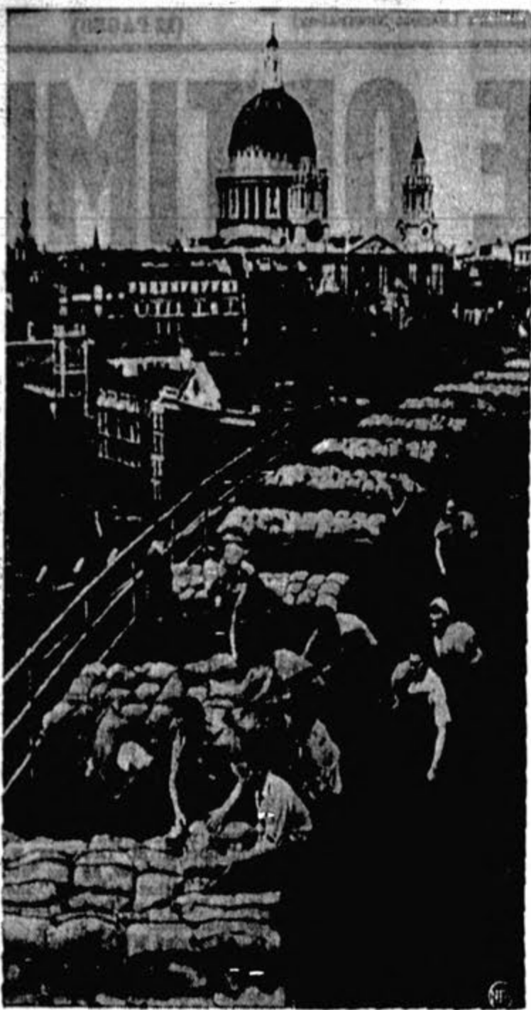
With all London furiously preparing for war, workers pile sandbags atop office buildings to provide protection against bombs. Dome of St. Paul's Cathedral, background, would make ace target for air raiders. (NEA Radiophoto)
