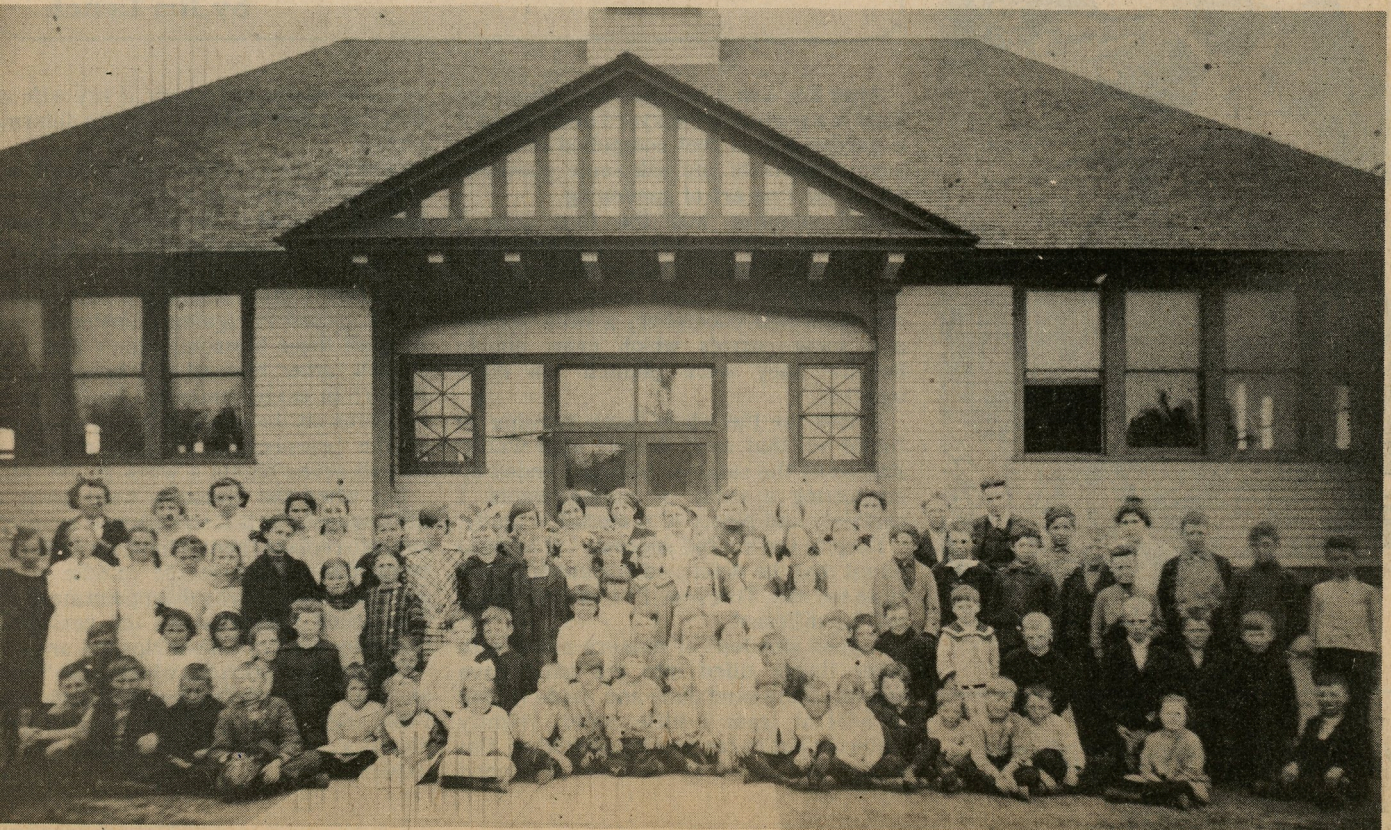
PICTURED ABOVE is the Thompson No. 1 School. The picture was taken around 1899 after the addition of two rooms was made.
