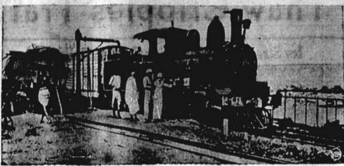
The French-owned rattletrap railway between Djibouti, French Somaliland, and Addis Ababa, Ethiopia, became a steel bone of contention between France and Italy as the latter agitated for important concessions. Above, an engine takes on water at Djibouti, seaport terminus.
