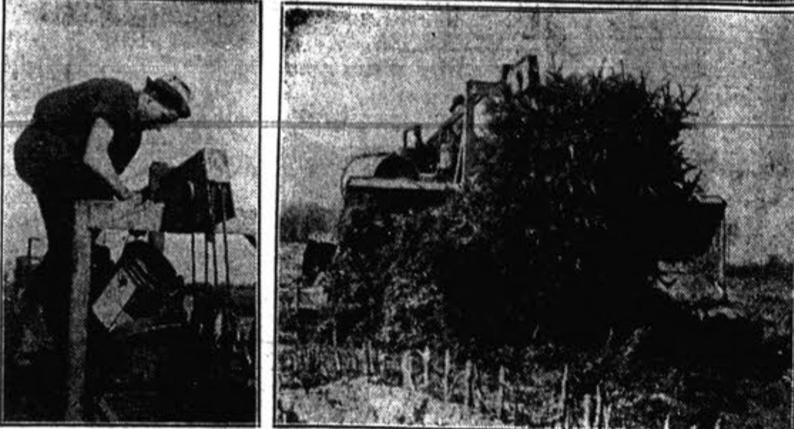
Clearing and leveling land presents no problem to the powerful bulldozer-equipped tractor shown above at work on the Sedenquist farm on old state road near Ford River. It is shown (top) leveling off a knoll and removing a stump at the same time, and (below) taking out a jackpine. Plenty of water is required by the tractor's cooling system (left). The machine is capable of uprooting large stumps and trees as well as leveling off rough spots on the fields.
