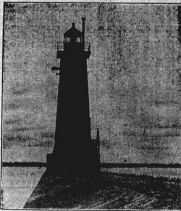
The Manistique lighthouse, pictured above, is located at the extreme end of the east breakwater. Unlike most lighthouses, however, nobody occupies it, as the equipment is operated by remote control from the lighthouse keeper's residence, several hundred yards away.
