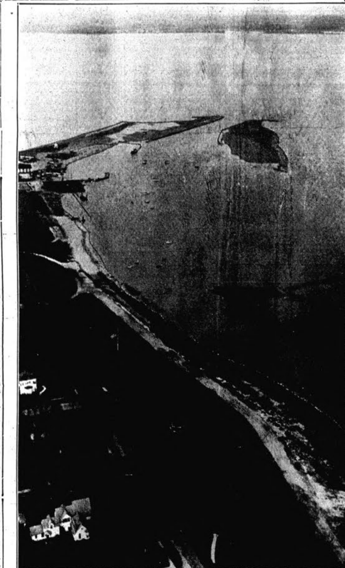
FROM THE WEST a recent aerial view of the yacht basin project shows the series of sand bars and weed beds at water level which will require little filling in to convert them into the arm of land that is to encircle the park lagoon for boating, canoeing and skating. These sand bars are to be built up with sand dredged from the yacht harbor basin and the lagoon in the center of the peninsula.
