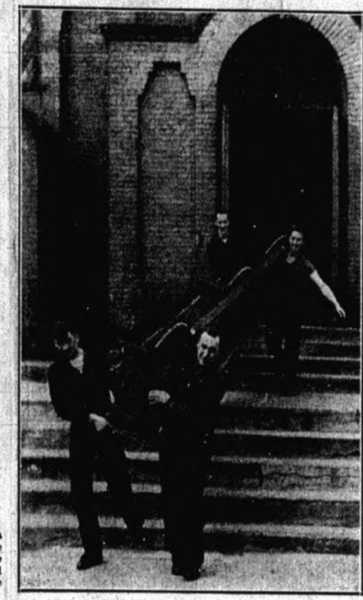
Members of the parish (right) started the task of razing the structure yesterday morning when they moved over 200 pews to the William Bonifas Memorial gymnasium where services will be held during construction.
