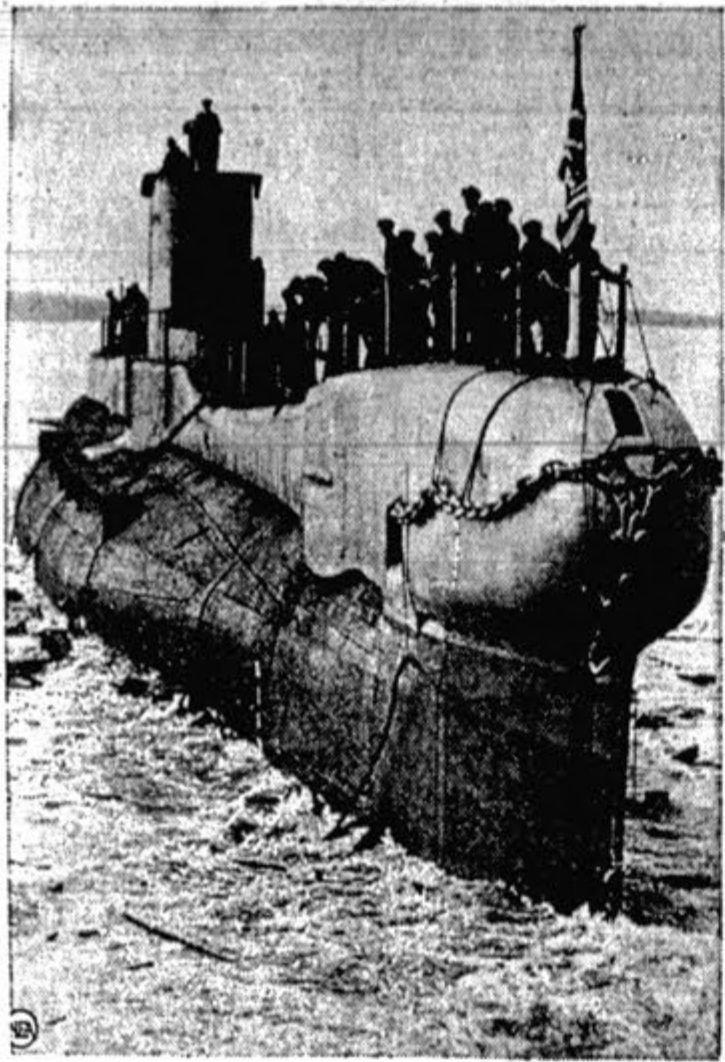
The new 1090-ton British submarine Triumph resembles some great monster of the deep as she slides into the water at Barrow-in-Furness, England. The Triumph carries a four-inch gun and six torpedo tubes. Launched along with the vessel at high tide were two smaller submarines designed especially for quick diving.
