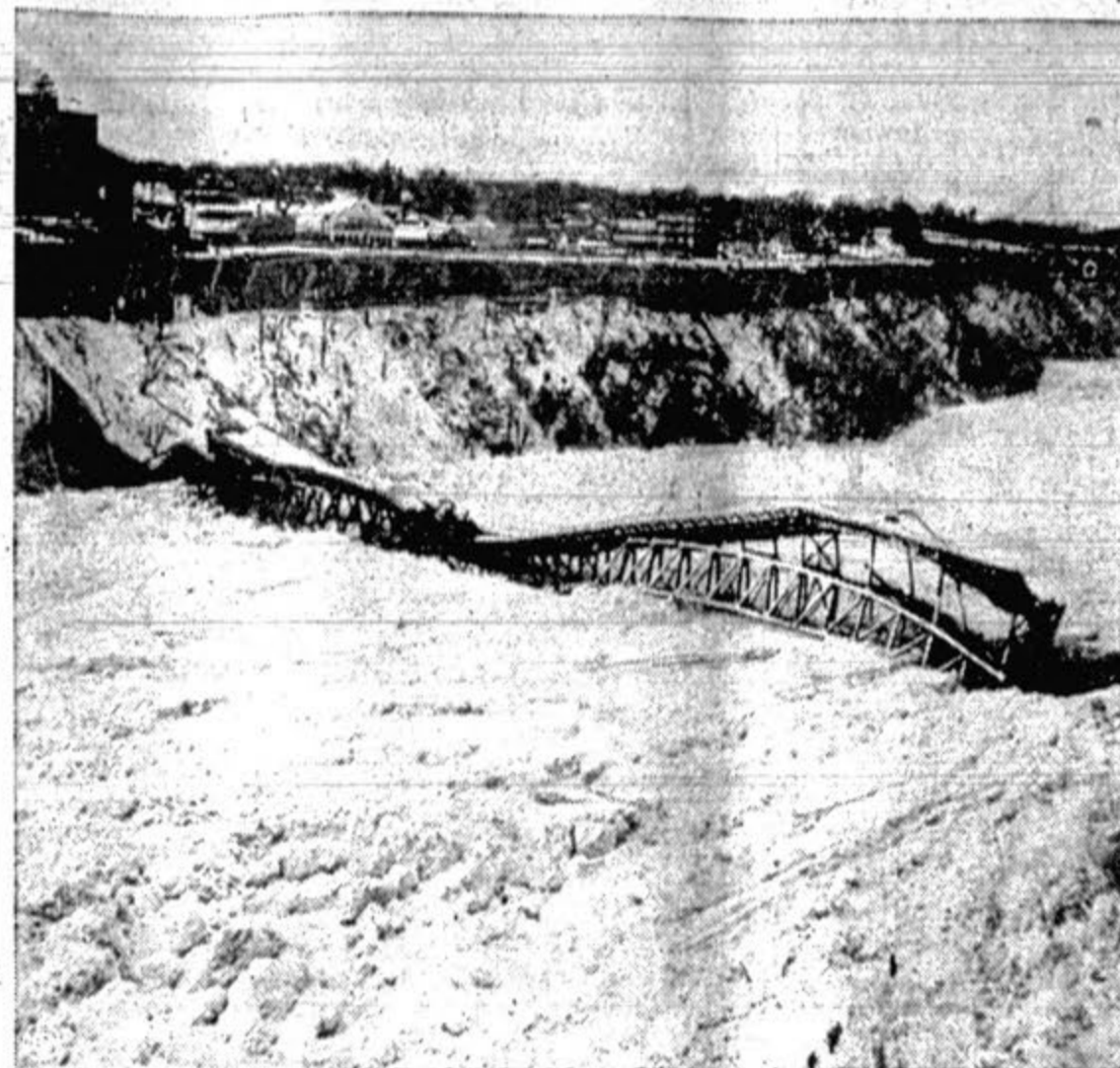
With a roar that drowned out Niagara itself, famed "Honeymoon Bridge" tore loose from its moorings on two nations and collapsed into the gorge of the Niagara river, missing the three workmen who appear as tiny dots at lower right. Losing a 36-hour battle with an ice jam 90 feet high, the historic steel span moved downstream slowly, a twisted ruin riding a modern "glacier."
