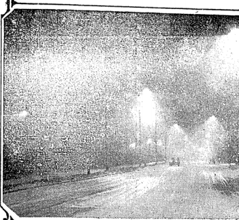
"SAFETY WITH LIGHT" installation, Washington Avenue, Saginaw, Mich., just in front of the Chevrolet foundry. Due to the particularly dangerous conditions at that point, the installation was made by the Consumers Power Company. (Right) Night Safety Analyzer.
