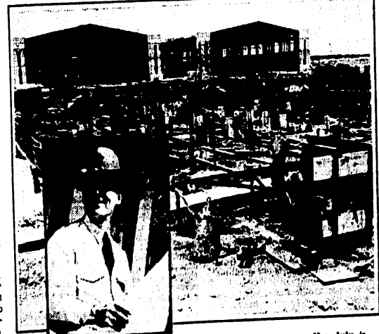
Construction of the huge new hangars at Hickam Field near Honolulu is going ahead steadily, with Capt. H. B. Nurse (above) in charge.
