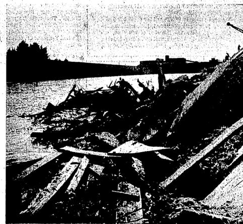
JUMBLE---Some of the debris and logs found in the bottom of the emptied flume can be seen in this view looking toward the mill.
