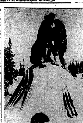
TESTING THE ROOF OF AN IGLOO—These soldiers of the U. S. Arctic Infantry patrol have completed a snow hut on the shores away up north and are making sure that the dome will withstand more than 500 pounds weight. These huts provide shelter for troops for many weeks.
