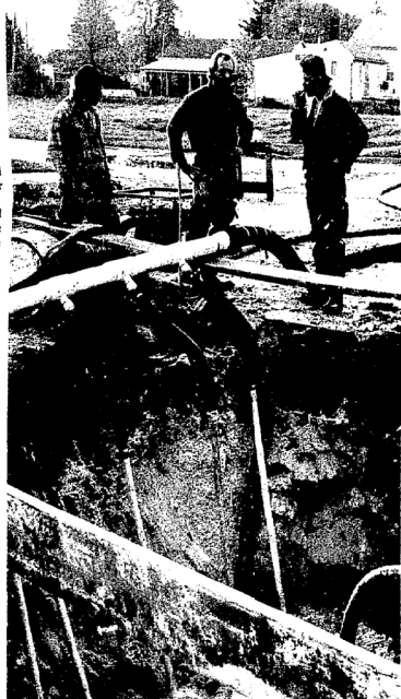
ANOTHER SEWER MAIN broke approve a $2.2 million bond issue in Manistique last week. This time Nov. 2 to separate-and replace the break occurred on M-94 and many sanitary and storm sewers in narrowed the highway to one lane the city. Sewer and water main while city workers dug down to the breaks have plagued the city for years. City voters will be asked to years.
