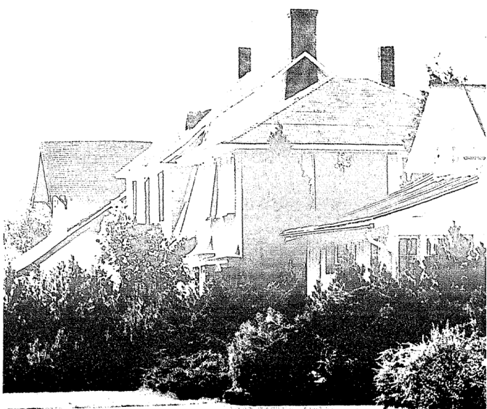
Say good-bye to US-2 HERE'S A VIEW that no one in Manistique will be able to enjoy again. This row of stately houses on west Arbutus has been torn down to make way for the rerouting of US-2 through the south side of town. State transportation department officials said that bids may be let for the project, which includes a four-lane bridge across the Manistique River, by December, with construction to begin as early as next spring.
