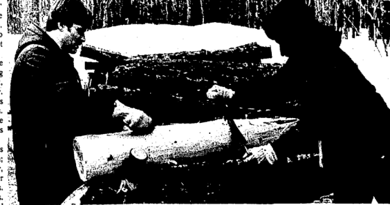
TWO CONVICTS from a work camp at Shingleton are among the crew of 10 that travels to Indian Lake State Park daily to help out in maintenance and construction work. These inmates are peeling the bark off a cedar post logged by the crew that will eventually be used as a sign post. (Gordon Archer photo)
