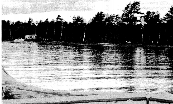
Pioneer Tribune photo: The emergency infrastructure repair under U.S. Highway 2 isn't the only surprise expense facing the city. A recent storm has caused damage to the boardwalk and threatened the shoreline campsites at the Manistique Lakeshore Campground. Pictured: As seen beyond the buckled and damaged boardwalk leading to the west breakwall, rocks are meticulously piled in front of a Manistique Lakeshore Campground site as most of the berm and shoreline in front of the campground washed away in the storm.
