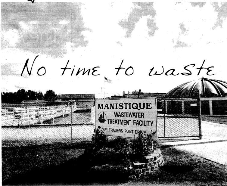
Above, the Manistique Wastewater Treatment Facility, along with the city's water plant, operations and projects were the focus of Monday's meeting of the Manistique City Council.
