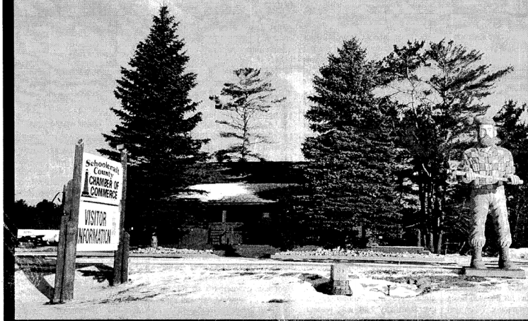
The former Schoolcraft County Chamber of Commerce building sits empty Wednesday morning, despite the recent flurry of activity and debate surrounding its sale to the city of Manistique.
