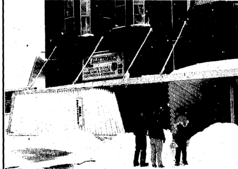
On Friday morning, the weight of accumulated snow caused the awning at M & L Electronics on South Cedar Street to collapse. (Pioneer-Tribune photos)
