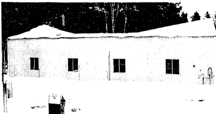
Left: an exterior view of the Big Bay de Noc School District bus garage after the roof collapsed sometime during the overnight hours Sunday into Monday. The garage was built in the early 1970s. (Pioneer-Tribune photo)
